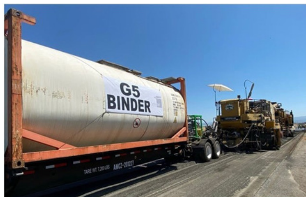
Image 3: G5 asphalt pavement binder from TechniSoil Industrial is made in part from discarded plastic bottles. Image provided by TechniSoil Industrial.
