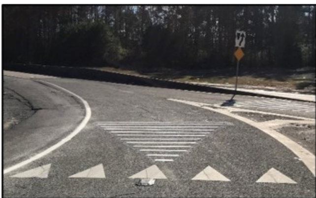
Image 6: Directional rumble strip pattern D3 installed in the field
