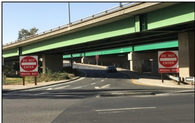
Image 5: Enlarged DO NOT ENTER and WRONG WAY signs
