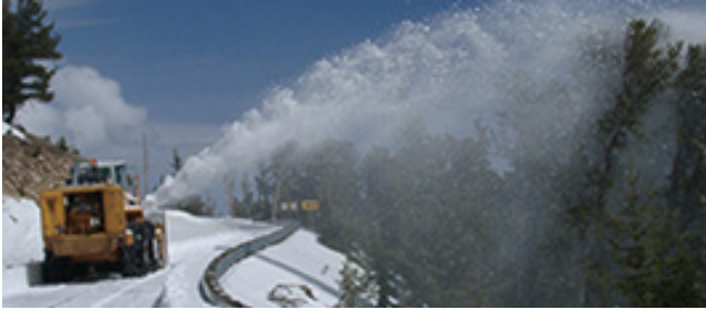
Image 1: Rotary blower removing snow from roadway
