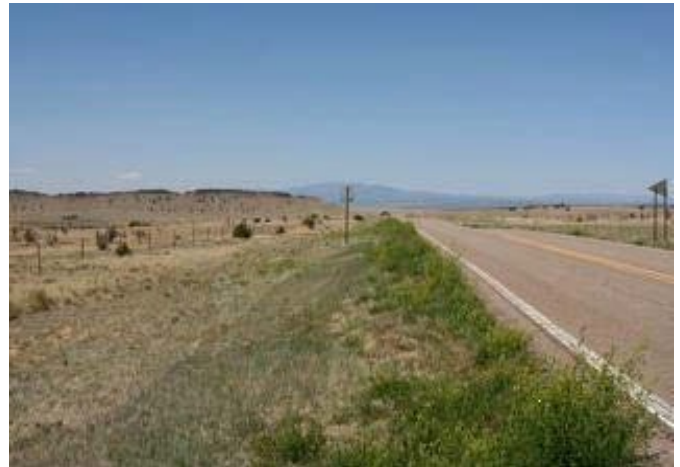
An example of the kind of native vegetation growing in the ROW that NMDOT will be quantifying to determine the amount of CO 2 that can be sequestered.
