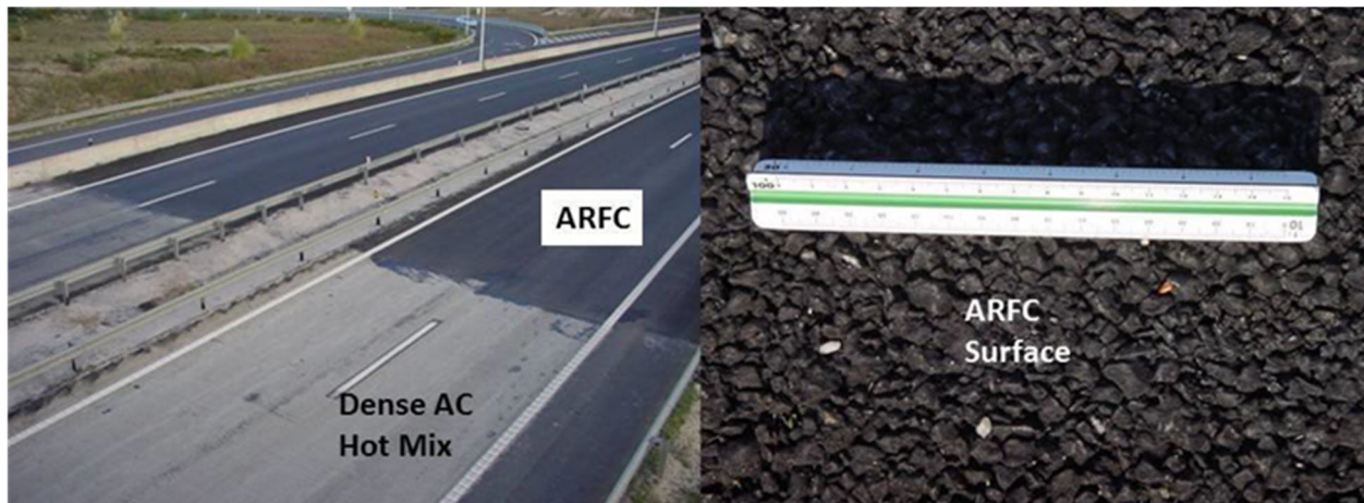
Figure 2.10: Dense-graded asphalt cement (AC) hot mix and asphalt rubber open-graded friction course (ARFC) surfaces in Portugal.
