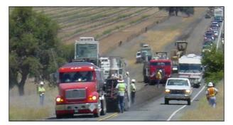
Figure 6.1: Pilot car traffic control on FDR project.
