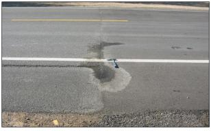
Figure 2.29: Early failure in patch (note water pumping in join).
