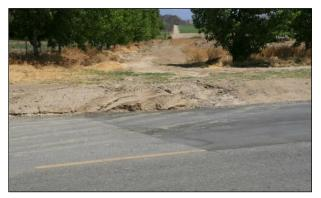
Figure 2.2: Example road below natural ground level.
