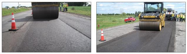
Figure 6.84: Primary compaction starting with smooth-drum roller on a PDR project.
