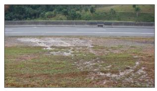
Figure 2.38: Water flowing downslope into the road.
