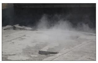
Figure 6.65: Pan after spreader has passed on an FDR-C project (4% stabilizer).
