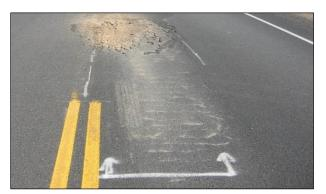
Figure 2.21: Example bottom-up distresses: Pumping of fines through cracks (a).
