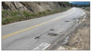
Figure 2.17: Example top-down distresses: Potholes.
