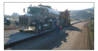
Figure 6.75: FDR-FA recycling train with no water tanker.
