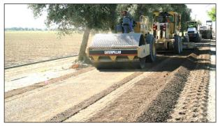
Figure 6.98: Final leveling and compaction interfering with primary compaction (FDR).
