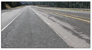
Figure 2.16: Example top-down distresses: Raveling.
