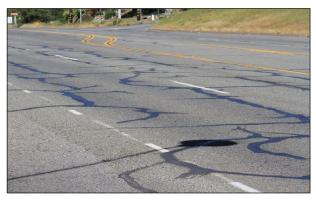
Figure 2.24: Example bottom-up distresses: Sealed reflective cracks.
