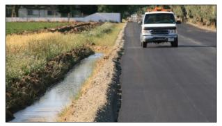
Figure 2.9: Example use of side drain to move irrigation water.
