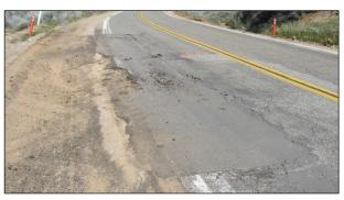
Figure 2.18: Example top-down distresses: Edgebreak.
