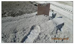
Figure 6.19: Accumulated cement dragged by hose at end of recycling run (FDR-C).
