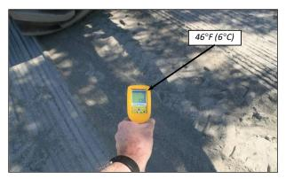
Figure 6.57: Active filler below specified starting temperature on an FDR-FA project.
