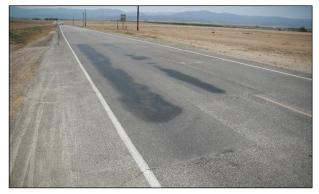
Figure 2.32: Bleeding in wheelpath repairs.
