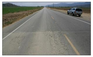
Figure 2.3: Example early full-width patch failure.
