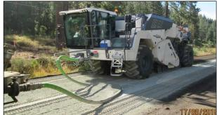
Figure 6.18: Recycler with no push bar and hose dragging cement stabilizer (FDR-C).
