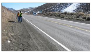
Figure 2.37: Absence of drains below cut slopes.
