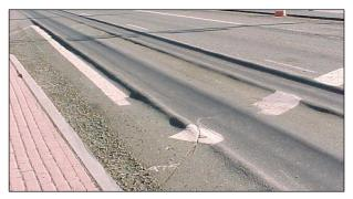
Figure 2.14: Example top-down distresses: Surface ruts during high temperatures.
