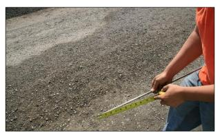
Figure 6.30: Measuring recycling depth on the Tbar (FDR).
