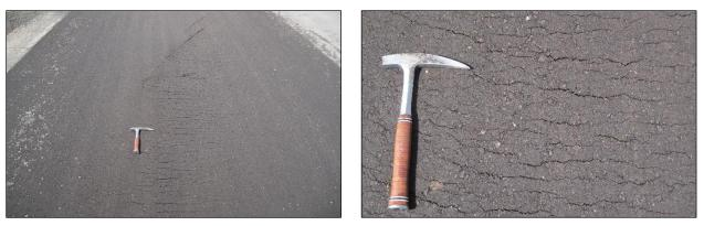
Figure 6.89: Shearing after completion of primary compaction on a PDR project.
