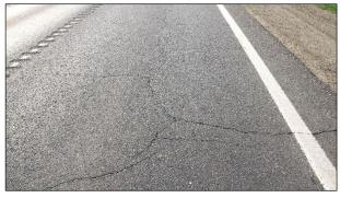
Figure 2.20: Example bottom-up distresses: Block cracks.
