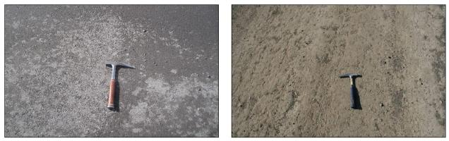
Figure 6.49: Good quality PDR and FDR surfaces after final compaction.
