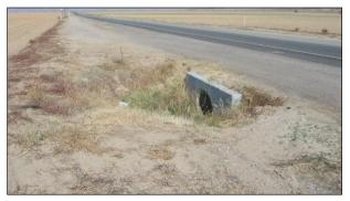
Figure 2.33: Blocked side drain and culvert.
