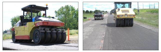
Figure 6.85: Primary compaction with pneumatic-tired roller on a PDR project.
