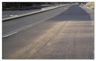
Figure 6.109: Curing seal after application of sand on a PDR project.
