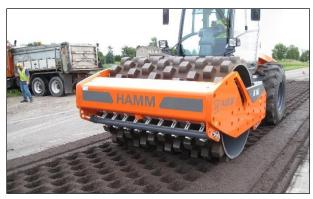
Figure 6.15: Vibratory padfoot roller on an FDR-FA layer.
