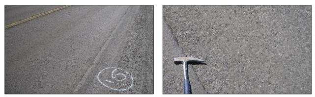
Figure 6.119: PDR layer milled for smoothness prior to placing asphalt concrete surface.
