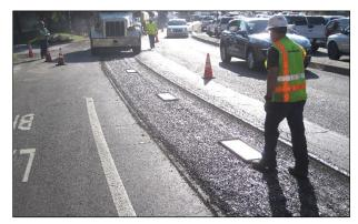
Figure 6.62: Placing active filler calibration pans on a premilled PDR project.
