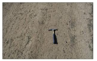
Figure 6.121: Acceptable surface prior to tack coat application.
