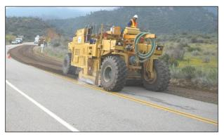
Figure 6.55: Prepulverization on an FDR project.
