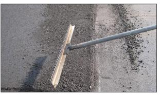
Figure 6.88: Raking to clear material and provide a sight line for the roller operator.
