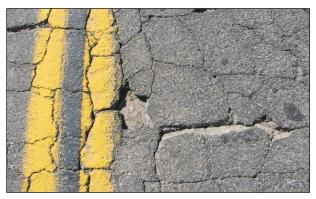
Figure 2.23: Example bottom-up distresses: Unsealed reflective cracks.
