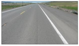
Figure 6.72: Reflected longitudinal crack in area of cement spread overlap (FDR-C).
