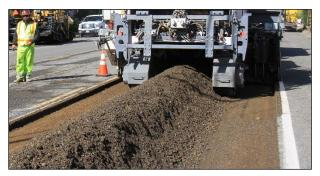
Figure 6.32: Good gradation and consistency behind the recycler on a PDR project.
