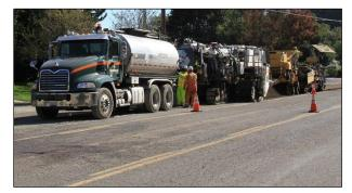
Figure 6.6: Single-unit PDR recycling train.
