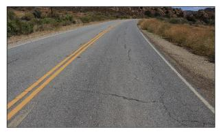
Figure 6.78: Early cracking caused by poor moisture distribution in recycled layer (FDR).
