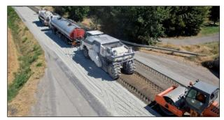
Figure 6.8: Wheel-driven FDR recycling train.
