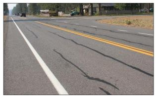
Figure 3.6: Alligator-A cracking on a PDR project.
