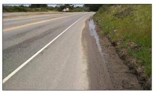
Figure 2.7: Example drainage problem in cut.
