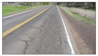
Figure 2.19: Example bottom-up distresses: Fatigue (alligator-B) cracks.
