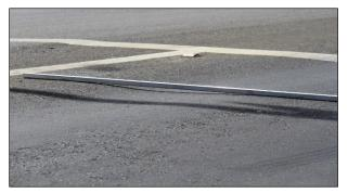
Figure 2.13: Example top-down distresses: Surface ruts/densification.
