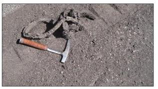
Figure 6.37: Crack seal behind the recycler on a PDR project.
