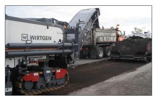
Figure 6.81: Removing excess material on a PDR project.
