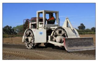
Figure 6.16: Segmented padfoot roller on an FDR-C layer.
