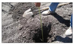
Figure 6.46: Checking recycling depth on an FDR-C project.
