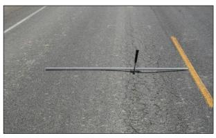
Figure 2.5: Example rutting associated with base/subgrade failure.
