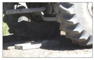
Figure 6.63: Spreader passing over pan on a prepulverized FDR-C project.
