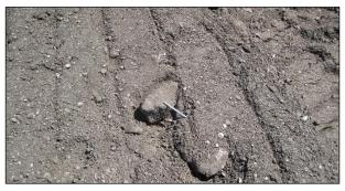
Figure 6.33: Oversize material behind the recycler on an FDR project.
