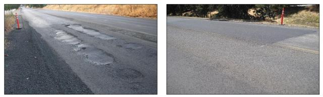
Figure 6.120: Patched distressed areas prior to surfacing.
