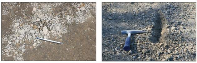
Figure 6.101: Segregation after excessive movement of material with a grader (FDR).
