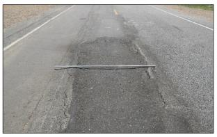
Figure 2.26: Example bottom-up distresses: Ruts associated with subgrade failure (b).
