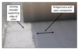
Figure 6.86: Roller bridging during primary compaction.
