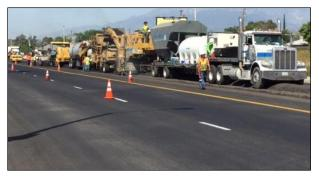
Figure 1.4: Partial-depth recycling train (multiunit).
