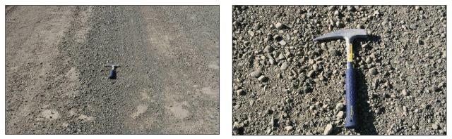
Figure 6.50: Unacceptable PDR and FDR surfaces after final compaction.
