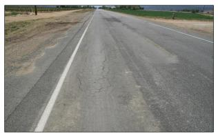
Figure 2.31: Early failure in wheelpath repairs.
