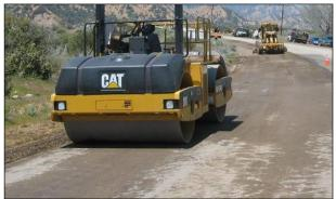
Figure 6.104: Intermediate rolling on FDR layer with double drum steel roller.
