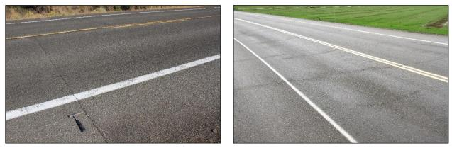
Figure 3.7: Reflected shrinkage cracks on FDR-C projects.
