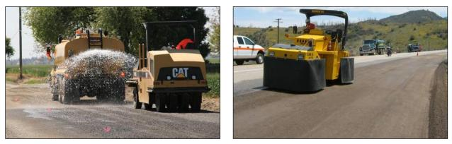
Figure 6.106: Final rolling on FDR projects with pneumatic-tired rollers.
