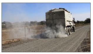
Figure 6.12: Active filler/stabilizer spreader.
