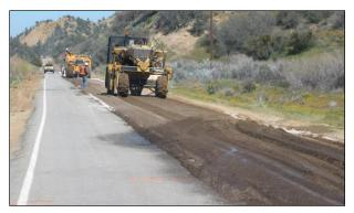
Figure 6.77: Water application between recycler and primary compaction roller (FDR).
