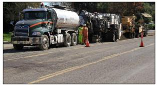
Figure 1.3: Partial-depth recycling train (single unit).
