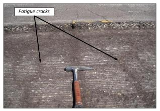
Figure 6.54: Fatigue cracks in underlying layer on a PDR project.
