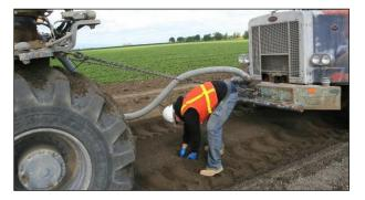
Figure 6.34: Sampling to check material consistency and gradation (FDR). (Note that working between the recycler and a towed vehicle is not recommended for safety reasons).
