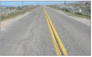
Figure 2.4: Example alligator-B cracking.
