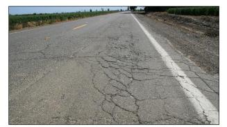
Figure 6.4: Distressed road prior to addition of new layer.
