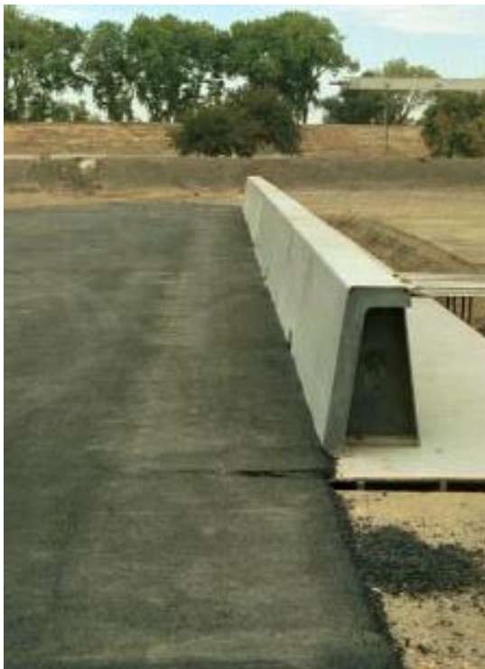
Figure 2-5. Type 732S test article after installation of the asphalt concrete overlay.
