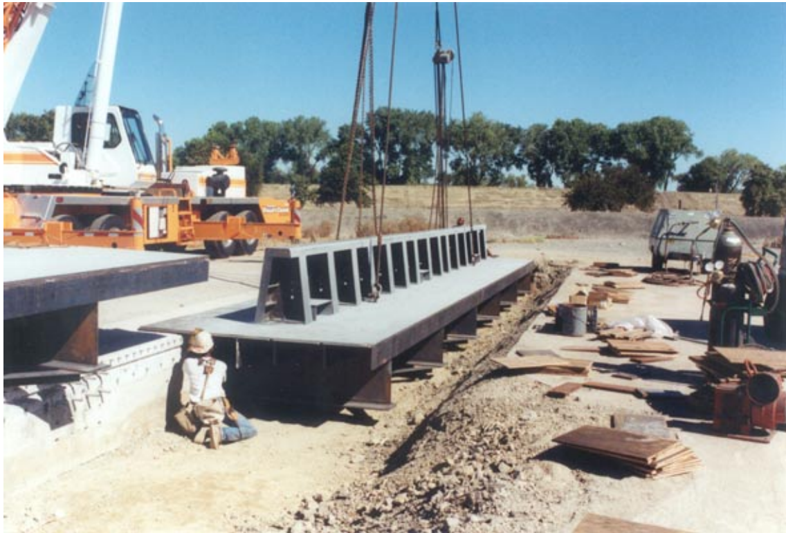
Figure 2-1 Type 732S barrier installation.
