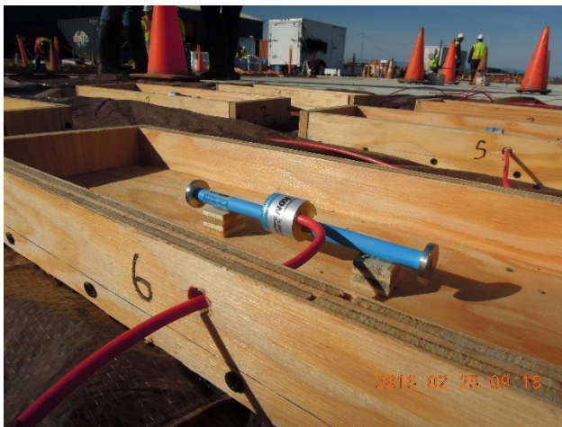
VWSG inside the mold
