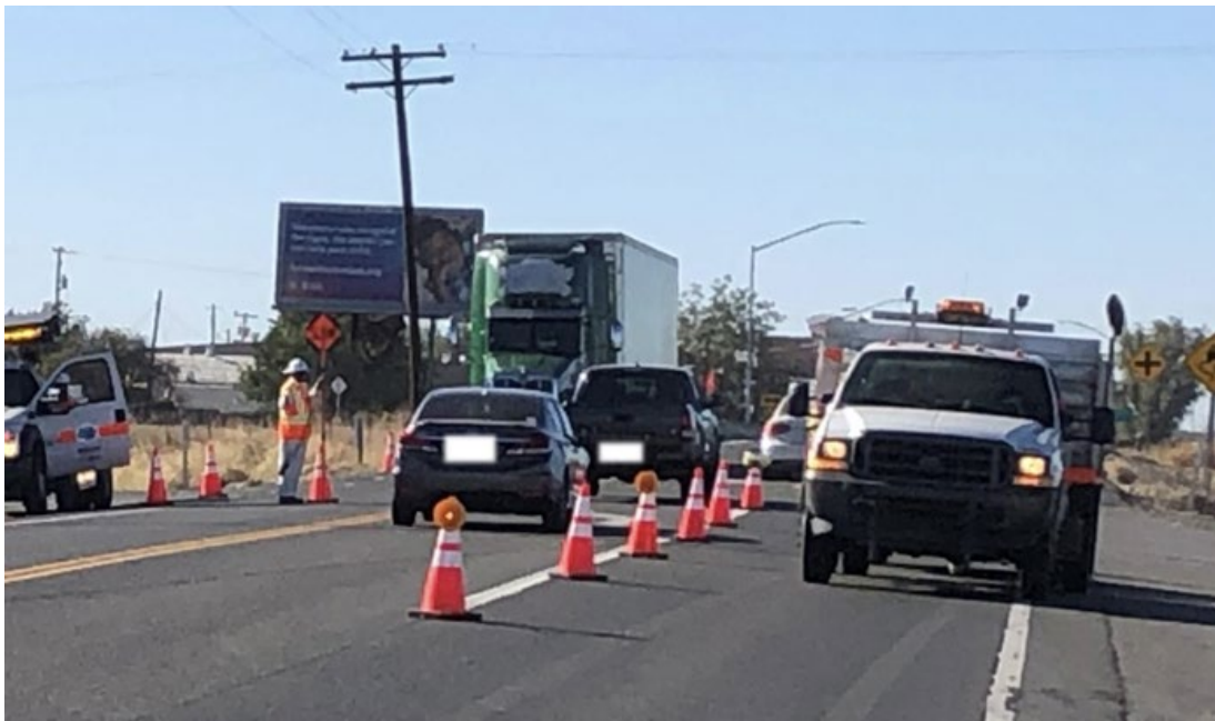
Figure 5.23 Deployment of Intellicone Lamps in Active Work Zone on CA Highway 113
