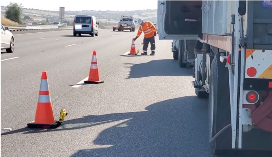
Figure 5.11 Maintenance Worker Deployment of SonoBlaster in Work Zone
