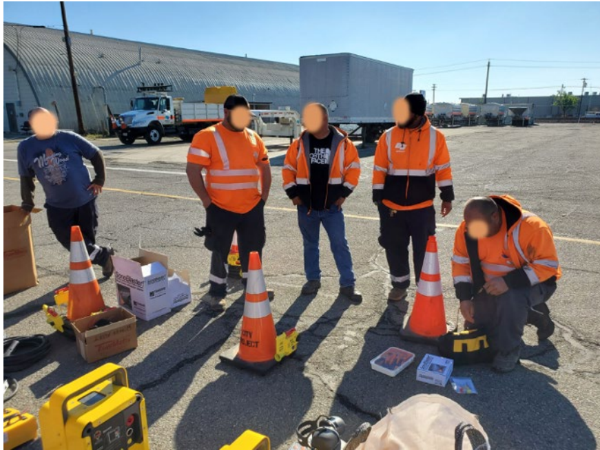
Figure 4.5 Crew Members Installing the SonoBlaster Unit
