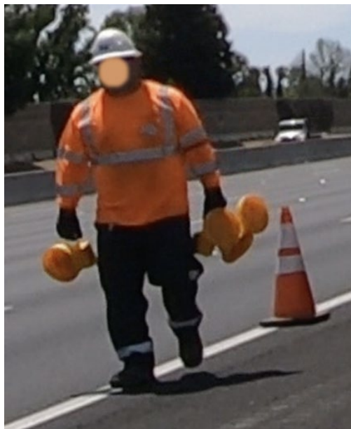
Figure 5.8 Retrieval of Intellicone Lamps by Maintenance Worker
