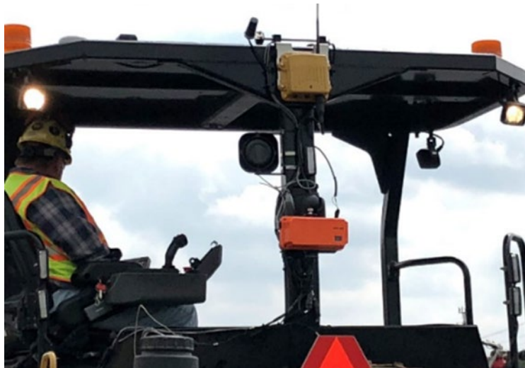
Figure 2.17 AWARE System Sensor Placement on Work Zone Equipment
