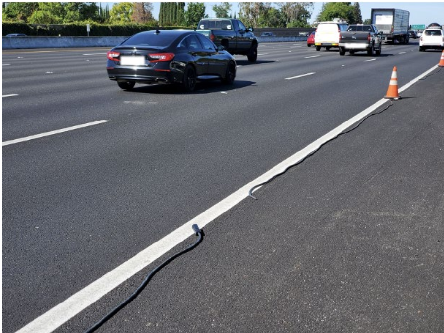
Figure 5.2 Placement of WAS Pneumatic Hose
