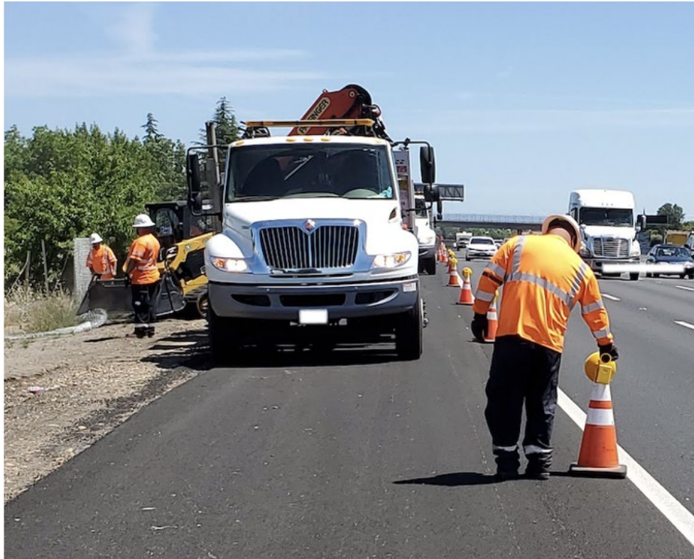
Figure 5.5 Deployment of Intellicone Lamps by Maintenance Worker
