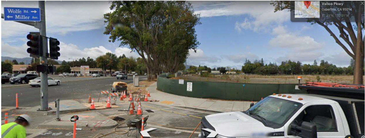
Figure 9.2. Wolfe Road and Miller Avenue, Vallco site under construction (Google Earth, 3/21/2021)
