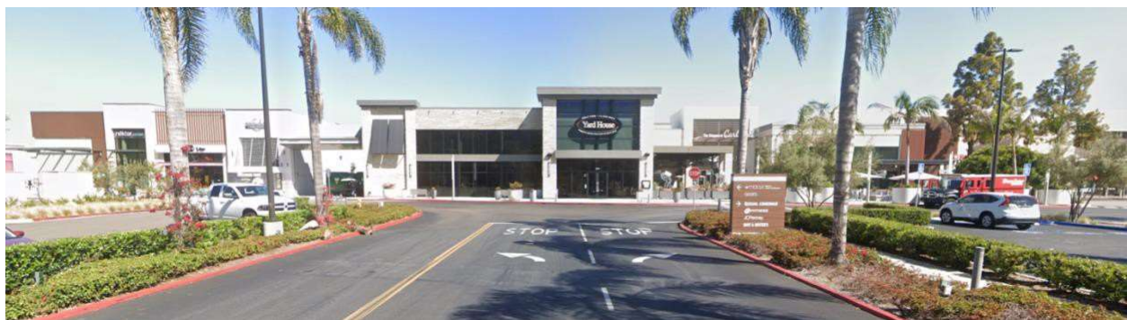
Figure 6.3. Entrance to the Shoppes at Carlsbad (Google Earth, 2/12/2021)
