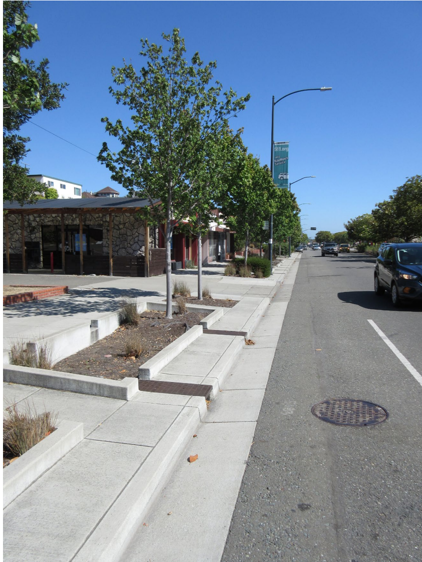
Figure 4. New Biostrips with Street Trees Provide a Pedestrian “Buffer” from Street Traffic on the East Side of San Pablo Avenue (Looking South) in El Cerrito, CA
