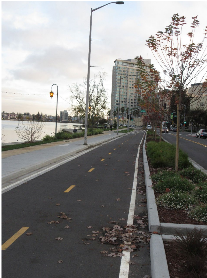
Figure 32. Looking South on Lakeside Drive in Oakland, in the foreground, the sidewalk is adjacent to the bikeway, and both are separated from traffic lanes by a planter strip with trees on the right. In the distant background, a segment with a biostrip between the sidewalk and bikeway can also be seen.
