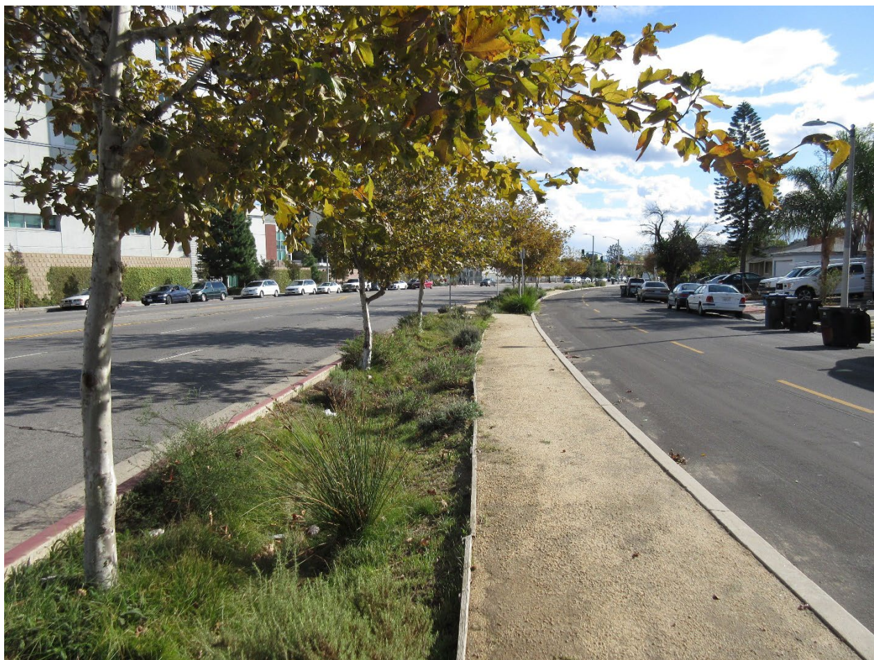
Figure 12. Looking South on Woodman Avenue, the frontage road on the west side (right side of picture) of the street is separated from the east side (arterial) by elevated and planted median with a meandering pedestrian path on Woodman Avenue between Saticoy Street to Lanark Street
