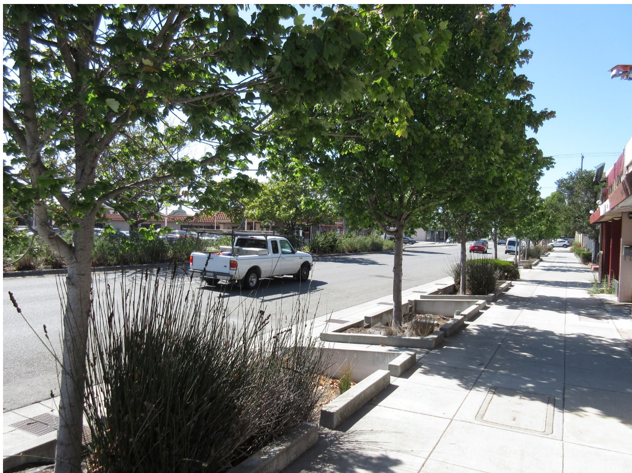
Figure 2. Recently Installed Elm Trees and Biostrips Along the East Side of San Pablo Avenue Between Lincoln Avenue to Eureka Avenue Looking North in El Cerrito, CA
