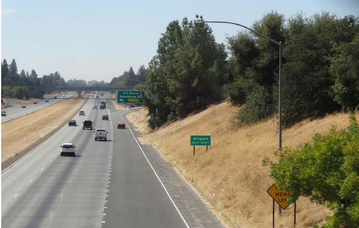
Figure 5.7 Below-grade cut section of SR 113 mowed by Woodland crew
