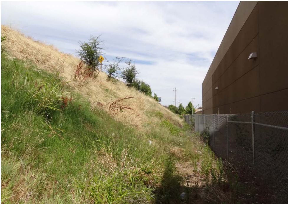
Figure 4.12: Slope measuring nearly 1:1 ( 45^\circ ) (SR 50 and 65 th St, SE quadrant) next to a commercial property
