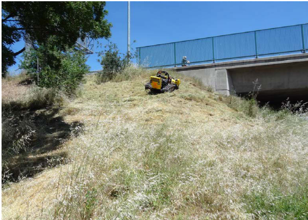
Figure 4.2: Traxx on slope transition from 2:1 (27°) to 1.5:1 (34°) under roadway
