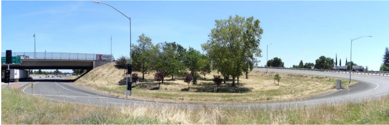
Figure 4.4: Landscaped area mowed with Traxx (SR 50 & Watt, SW quadrant)
