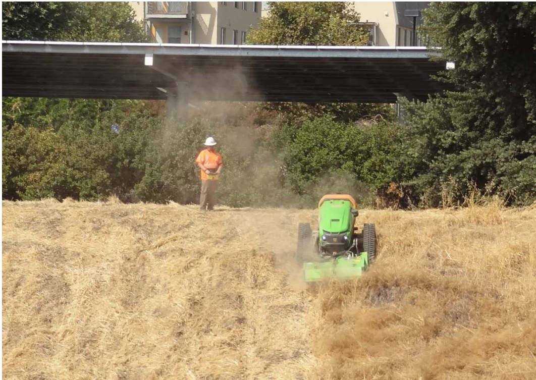
Figure 5.8 Mowing downward from top of slope
