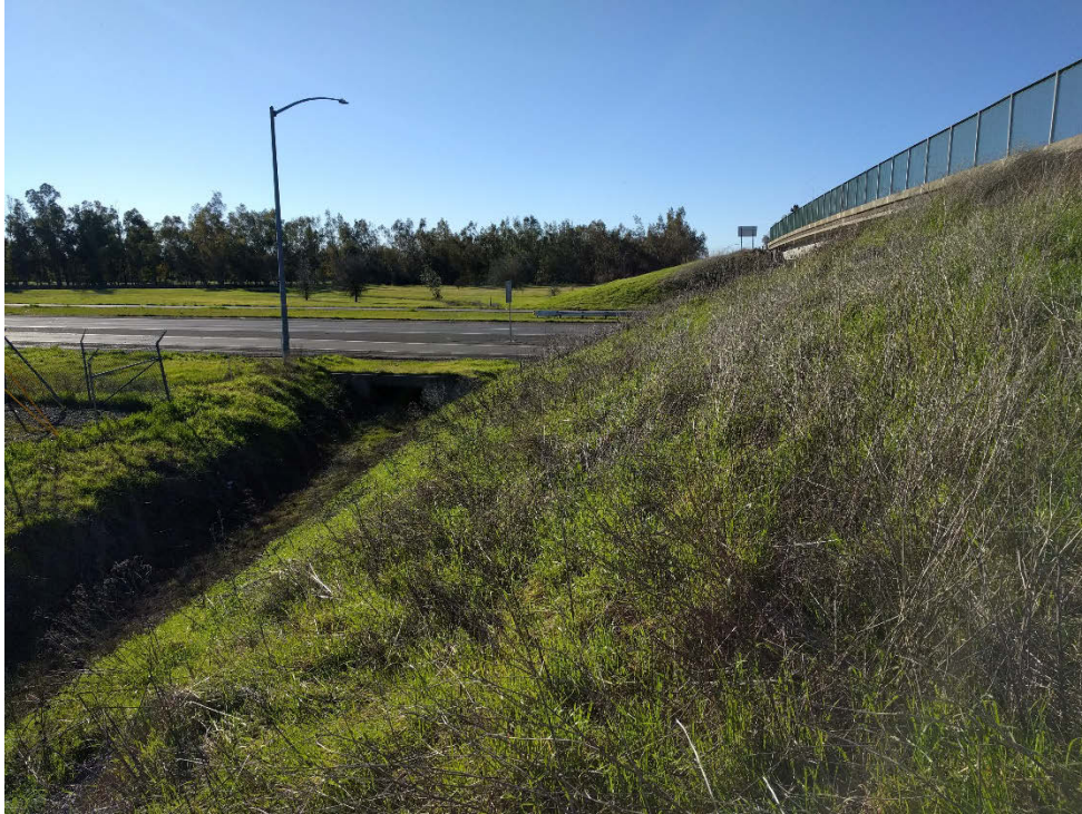
Figure 4.13: Slopes 1:1 (45°) in drainage (SR 113 and County Road 29 SE quadrant)
