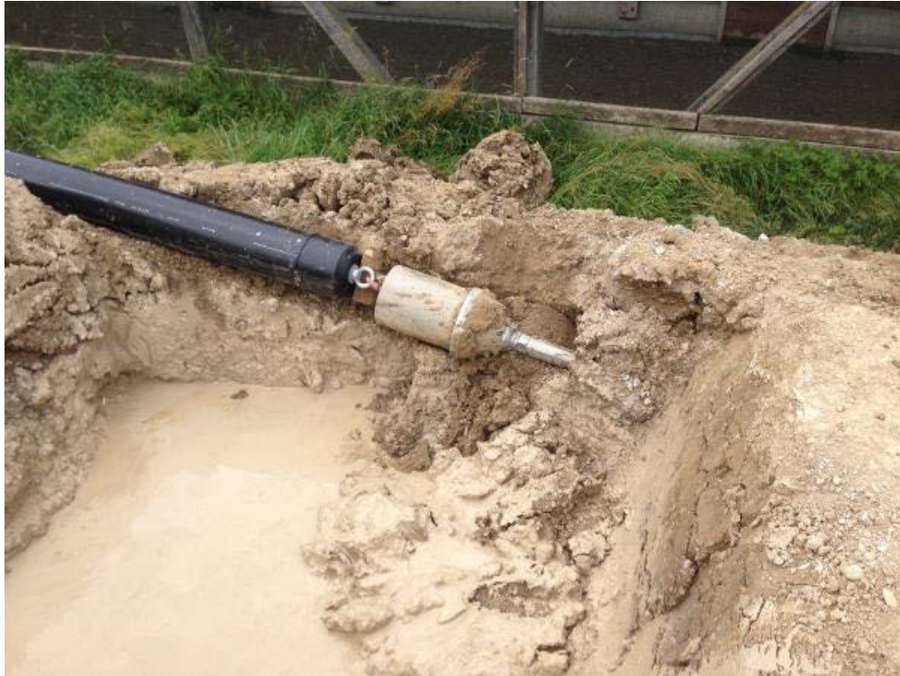
Figure 31: Pipe pulling (Source: Terra, Trenchless Technologies, 2018)
