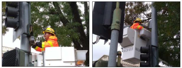
(c) Drilling hole in the small wire box on the signal pole
