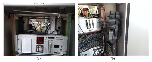
Figure 12 (a)-(b): Typical arrangement of the equipment housed inside the Signal Controller cabinet to provide power for the cameras and other devices
