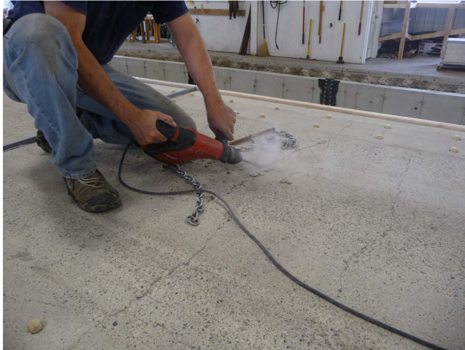
Figure 14: Removal of spalled concrete.
