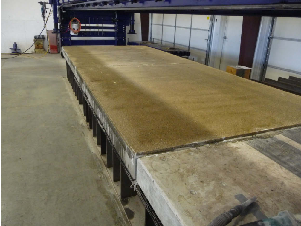
Figure 19: Final surface of polymer overlay.
