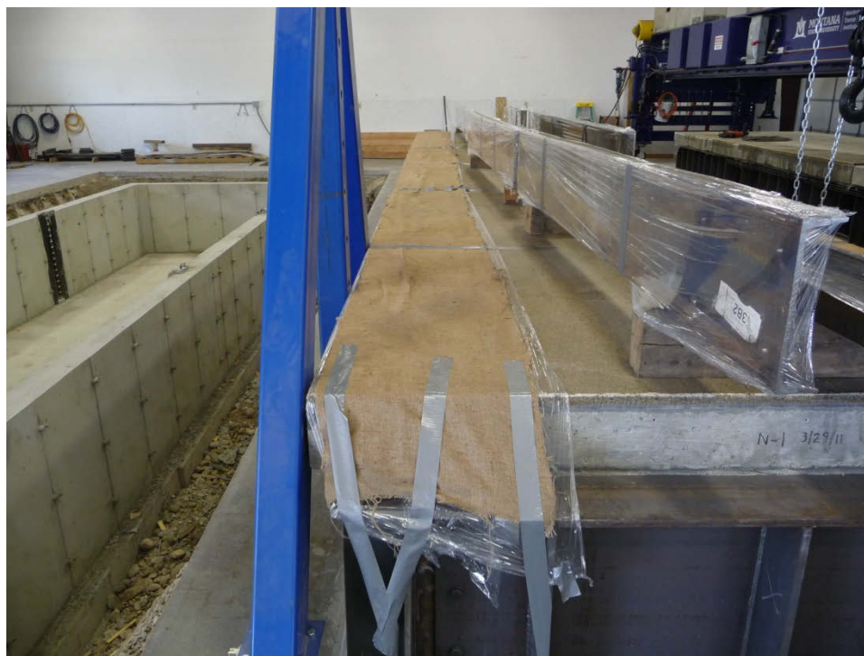
Figure 10: Burlap used to help spread grout on top of test panels.
