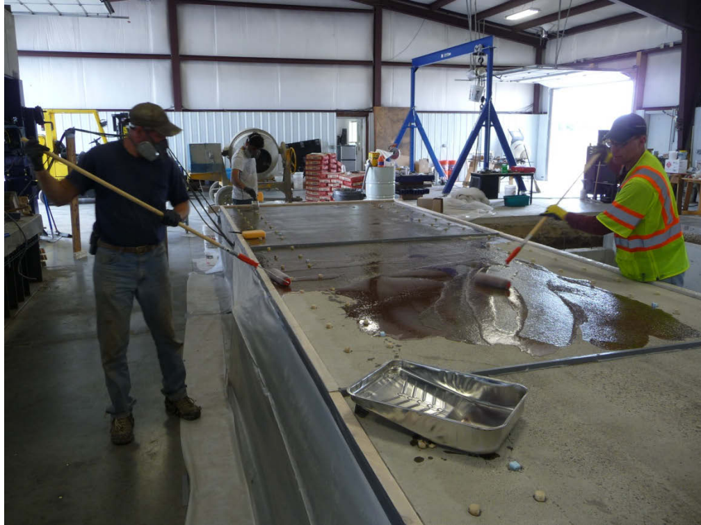
Figure 17: Application of HMWM surface treatment.
