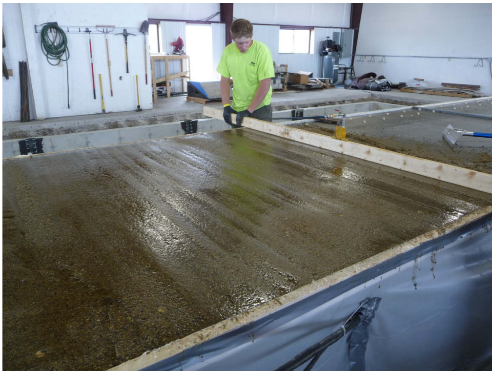
Figure 18: Screeding of polymer overlay.
