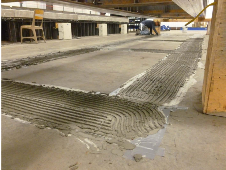
Figure 8: Grout spread on geosynthetic under elevated reaction frame.
