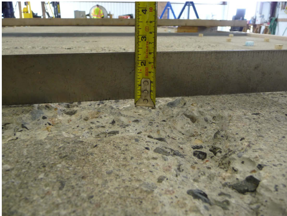
Figure 15: Typical depth of spalled concrete removal.
