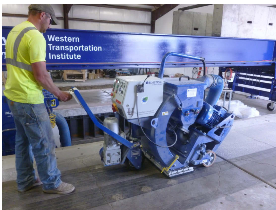
Figure 13: Shot blasting the deck panels in preparation for the polymer overlay.
