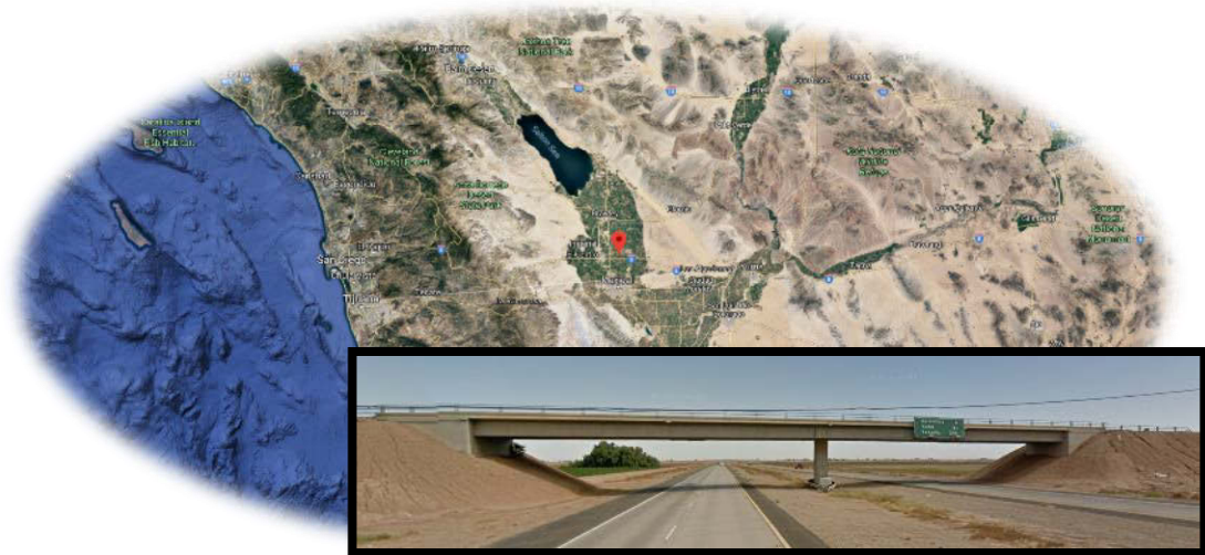
Figure 6-1: Meloland Road Overpass.
