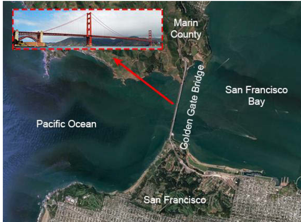
Figure 5-1: The Golden Gate Bridge.
