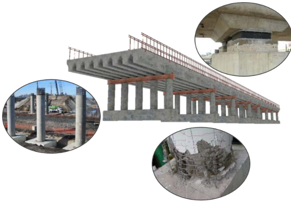
Figure 1-1: Major explicit sources of energy dissipation in bridge structures.
