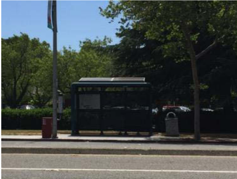
Figure 4-29 A typical stop with shelter
