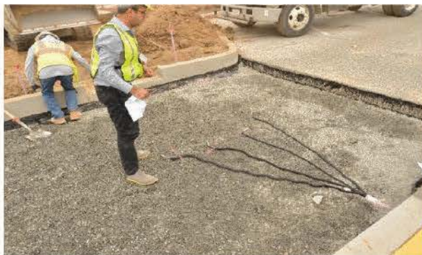
a) Placing strain gages
