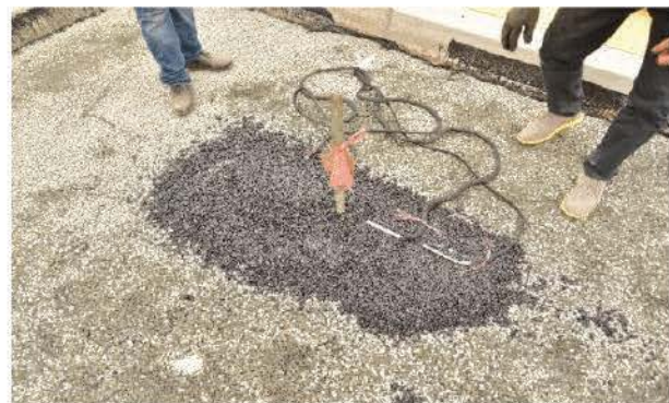
b) Placing strain gages on asphalt
