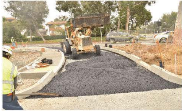
d) Pouring of HMA on test section
