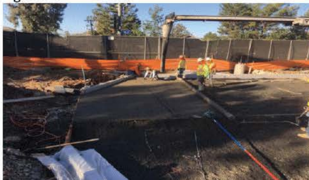
a) Permeable concrete placement
