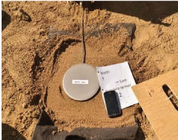
a) Installing pressure cell with directions
