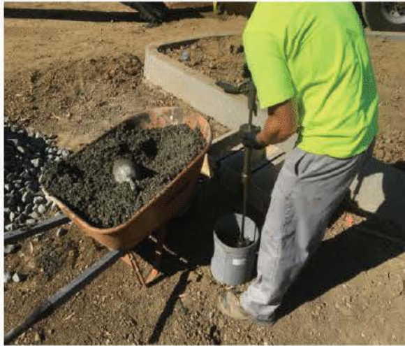
a) Compaction of sample
