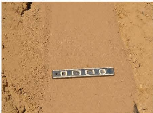
a) Leveling of subgrade
