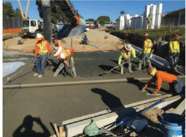
d) Compaction using hand floats
