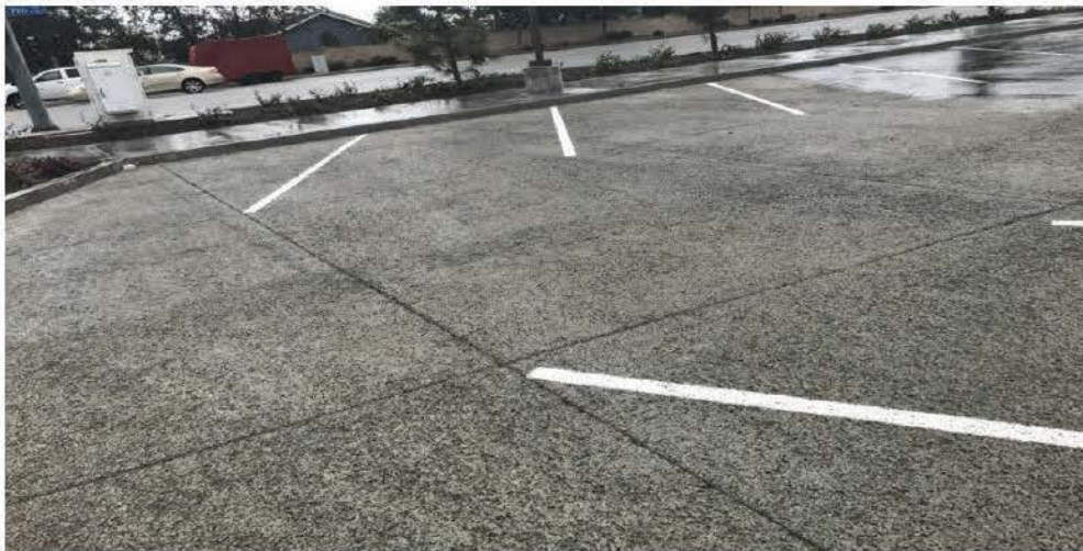
Figure 20. Fully permeable concrete pavement
