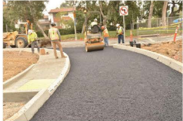
b) Compaction using static roller
