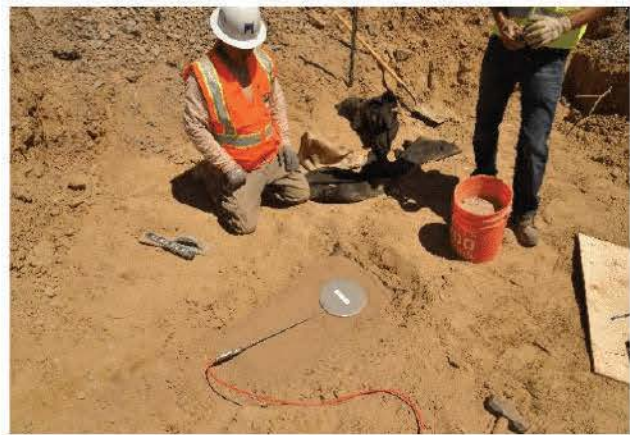
b) Installation of pressure cell
