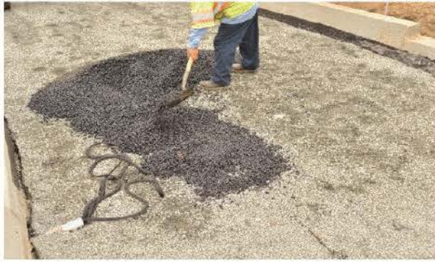
c) Pouring of HMA on strain gages
