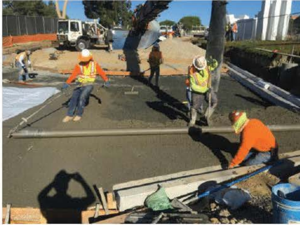
c) Compacting concrete using roller screed
