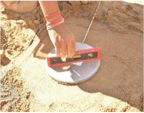
b) Leveling of pressure cell
