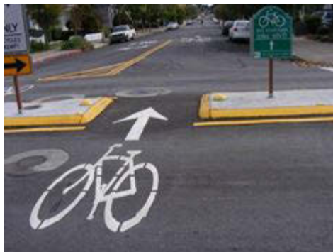
Figure 22. Median Cut Through for Bicycles
