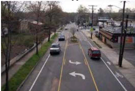
Two-way left turn lane
