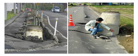
Fig. 4. Flotation of sewage line during the 2004 Chuetsu earthquake (after NISEE 2016).
