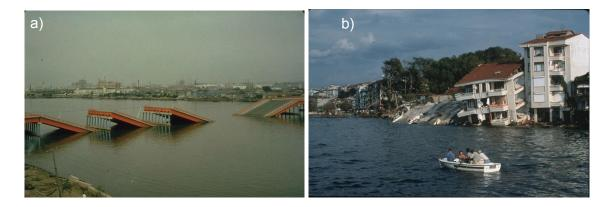
**Fig. 3.** a) Lateral spreading causing bridge spans to fall off from the supports during the 1964 Niigata earthquake, and b) Lateral spreading of waterfront properties during the 1999 Kocaeli earthquake (after NISEE 2016).
