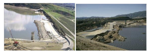
**Fig. 5.** Lower San Fernando Dam collapse due to San Fernando earthquake in 1971 (after NISEE 2016).
