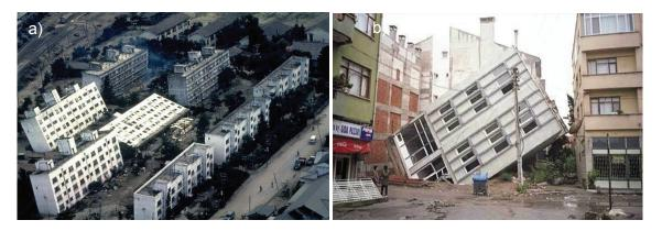
Fig. 2. a) Overturning failures in residential complex in 1964 Niigata earthquake, andb) Liquefaction-induced settlement due to loss of bearing capacity in 1999 Kocaeli earthquake (after NISEE 2016).
