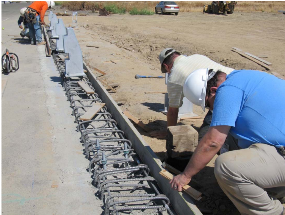
Figure 2-3 After the First Concrete Placement
