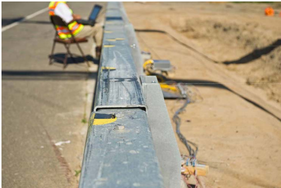
Figure 5-7 Test Article After Test 130MASH3P13-03 Close Up
