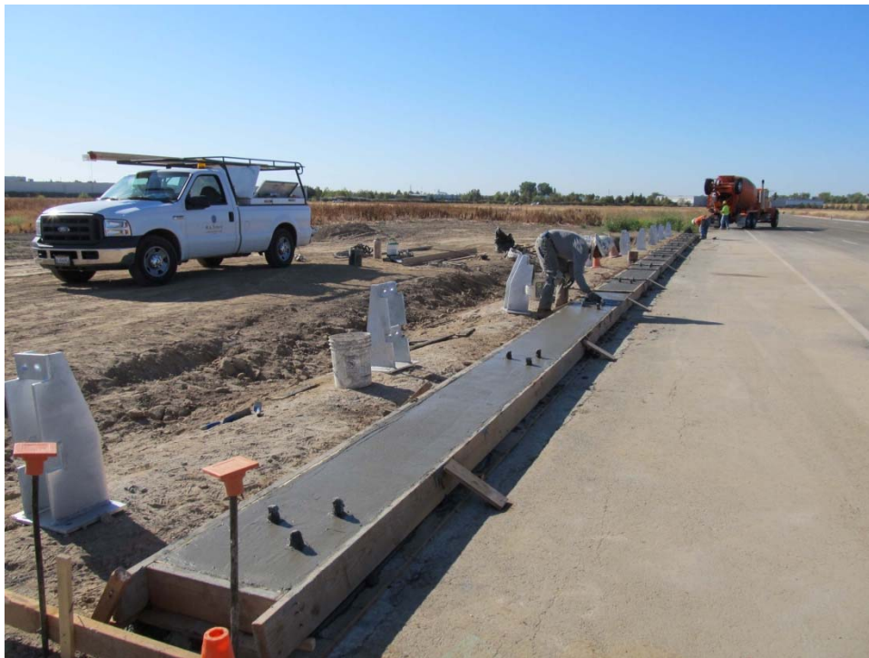
Figure 2-5 After the Second Concrete Placement
