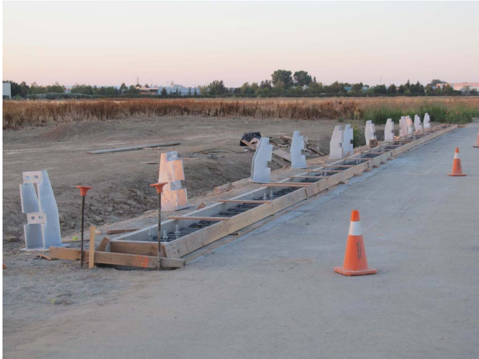
Figure 2-4 Before the Second Concrete Placement For Curb
