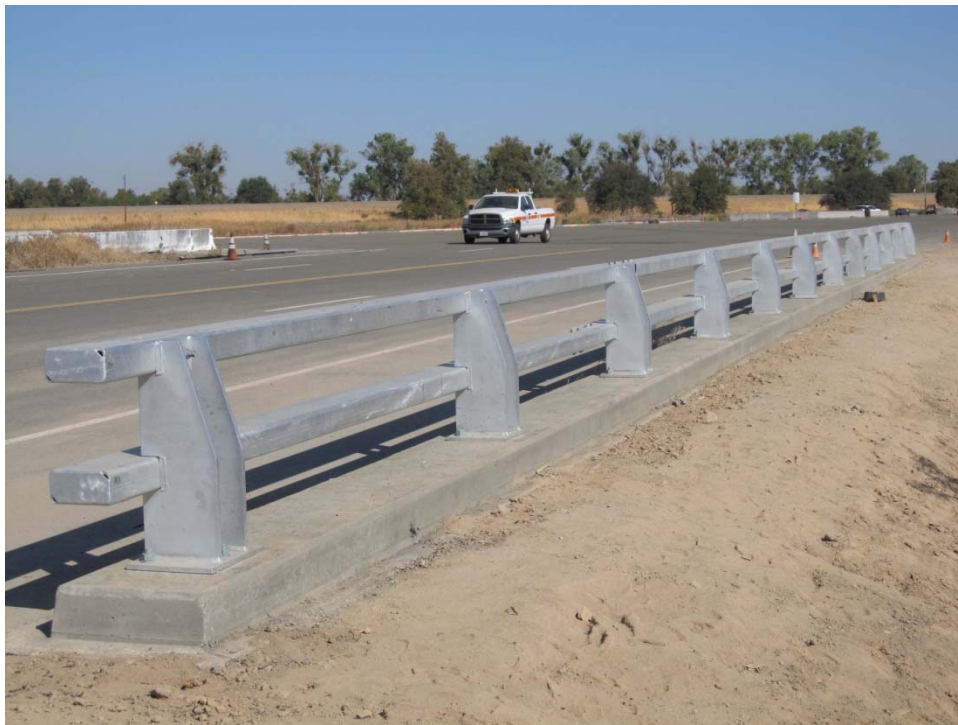
Figure 2-7 Completed Barrier Construction Back
