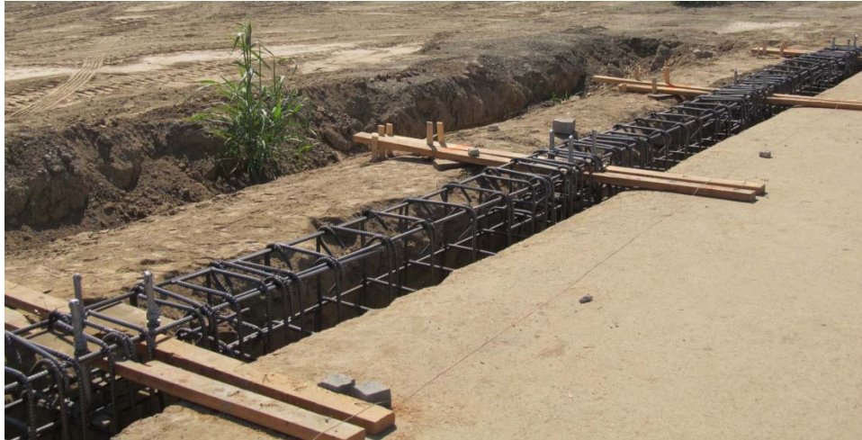
Figure 2-2 Rebar for Barrier
