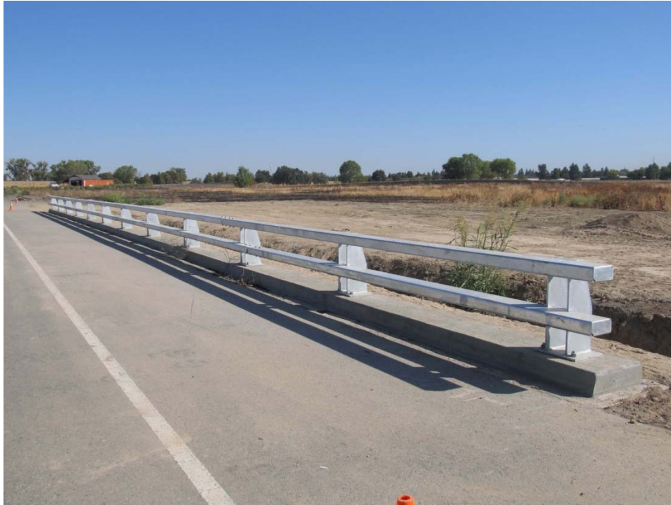
Figure 2-6 Completed Barrier Construction Front
