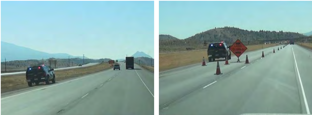
Figure 5. Locations of CHP vehicles: at the Beginning of Taper (left) and at the End of Taper (right).
