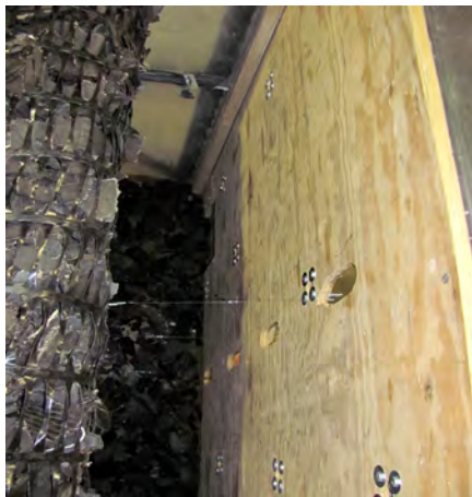
(a) TDA backfill
