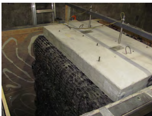
(a) TDA backfill
