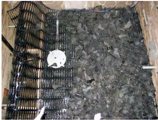
(a) TDA backfill
