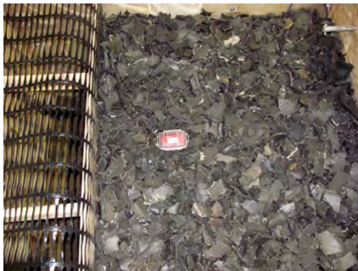
(a) TDA backfill
