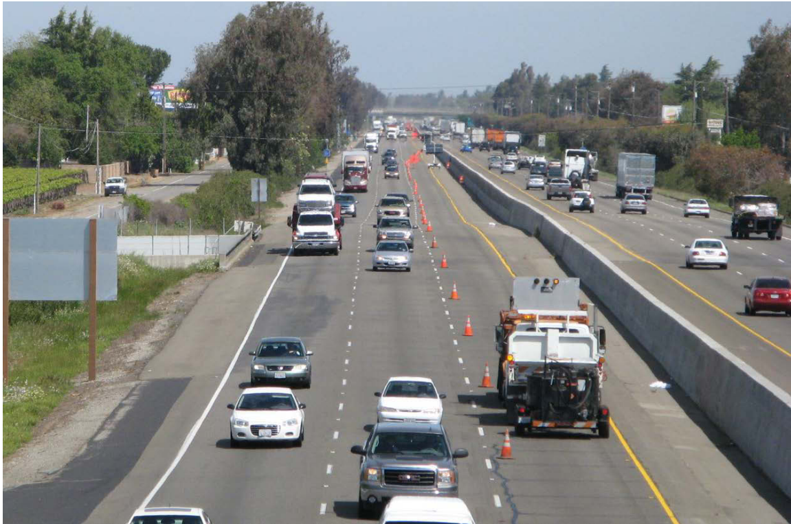
Figure 11: View Looking Down At the Test Work Zone of April 15, 2011.
