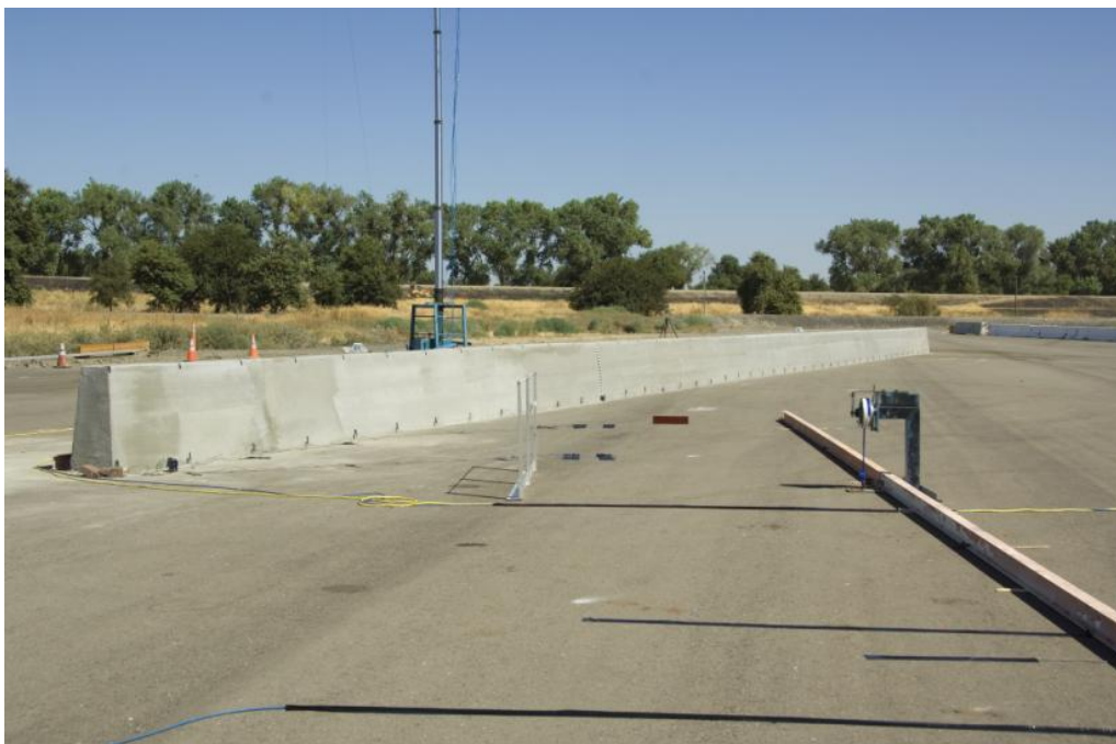
Figure 2-1 Type 60 Concrete Barrier Prior to Test
