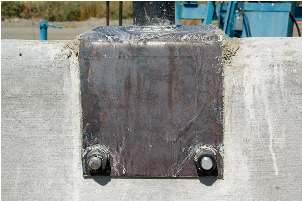
Figure 2-15 Signpost Saddle Prior to Test
