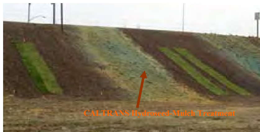
Figure 5.18 View of the Caltrans Hydroseed treatment on the highway fill-steep slope in November 2006.
