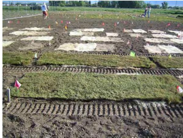
Figure 4.16 Installation of the four reinforcement materials: coconut-straw, jute, excelsior, and nylon netting (control) placed beneath the multispecies sod in Experiment B 2 (2007).
