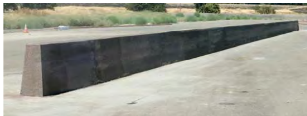
Figure 2-1 Type 60 Concrete Median Barrier
