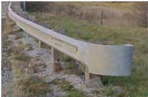
Figure 1-1 Breakaway Cable Terminal (BCT)
