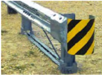
Figure 4-6 Six Post Slotted Rail Terminal (SKT-350™)
