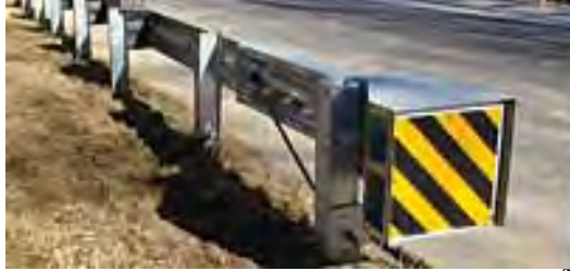
Figure 4-4 Sequential Kinking Terminal (SKT™)
