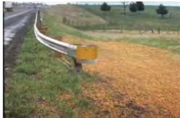
Figure 1-2 Modified Eccentric Loader Terminal (MELT)
