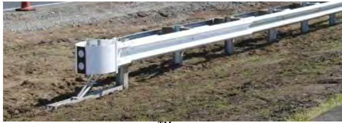
Figure 4-1 X-Tension™ Guardrail End Terminal
