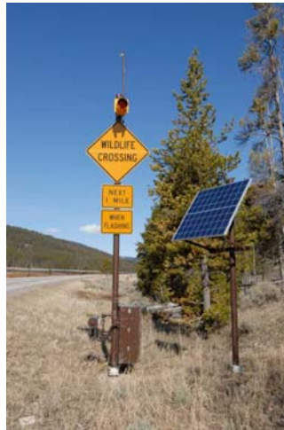
Photo 1. The animal detection system along US Hwy 191 in Yellowstone National Park (at mile marker 28-29) between West Yellowstone and Big Sky, MT (Photo: Marcel Huijser).
