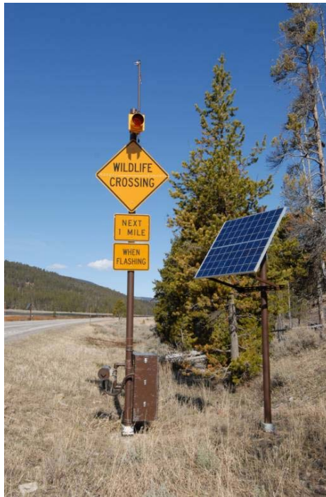
Figure 1.3: Activated warning sign (Beacon 1 for northbound traffic) with flashing beacon on top (Photo: Marcel Huijser, WTI-MSU)
