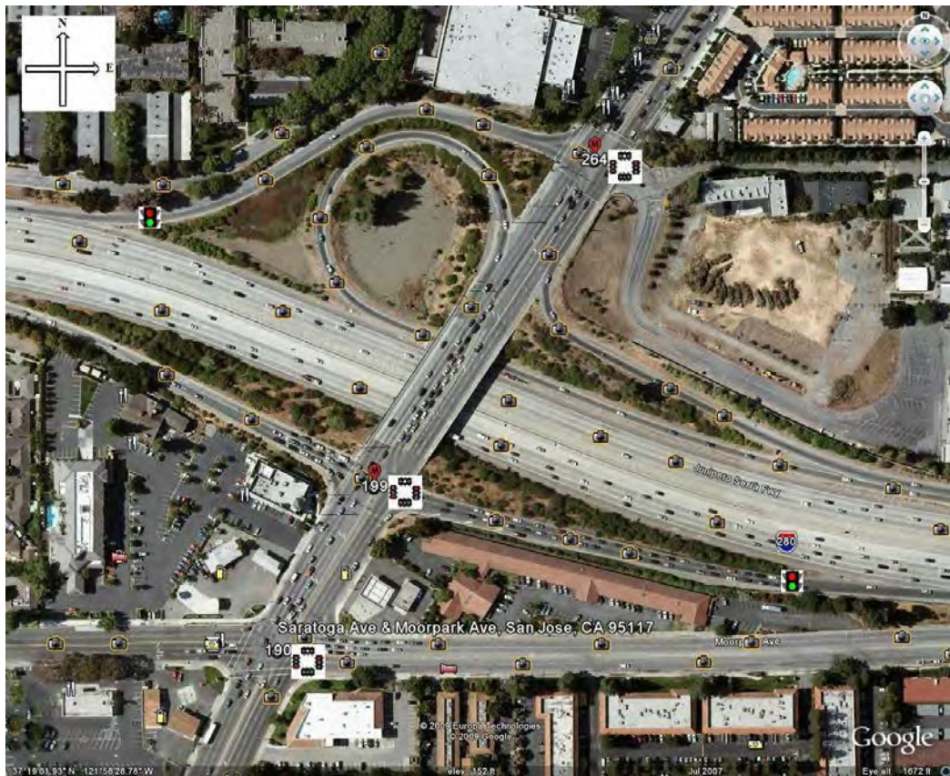
Figure A2-1. Road geometry with 3 intersection traffic controller and 2 entrance ramp meters;
