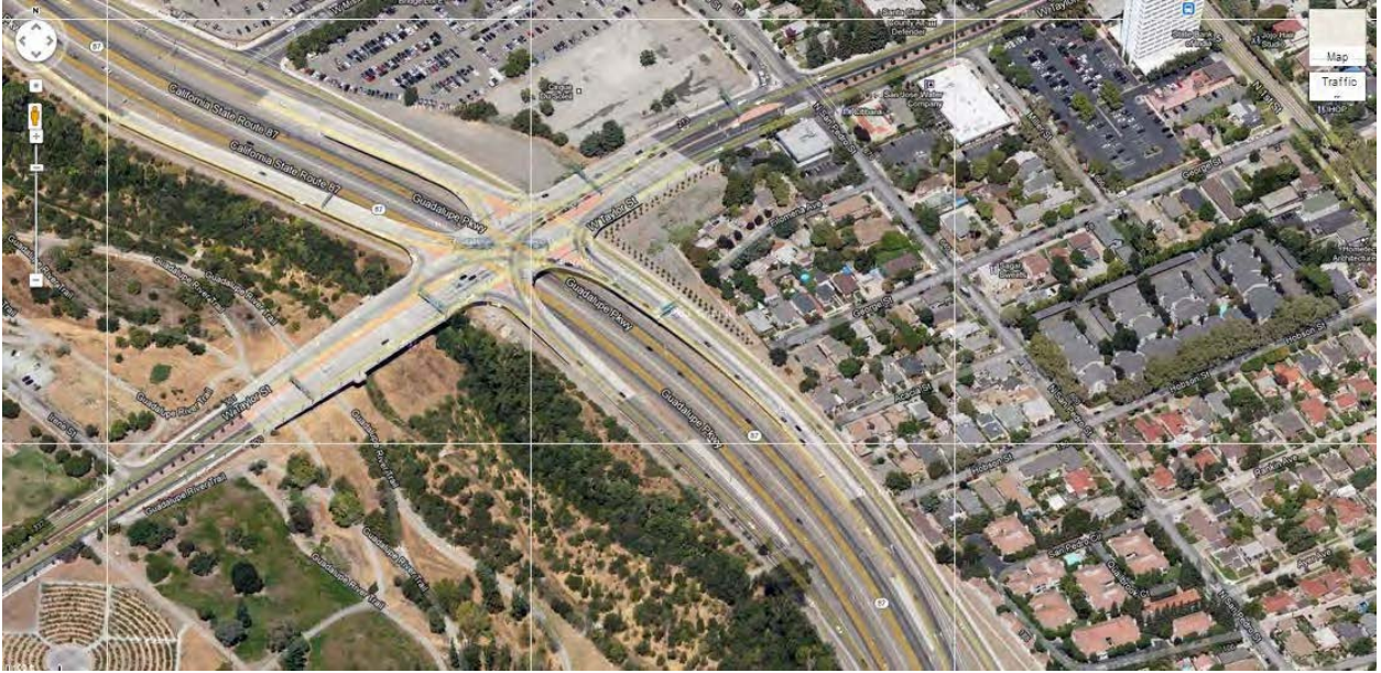
Figure 6-3. Overall road geometry of the system: (a) intersection at Taylor St., Intersection at San Pedro, and SB entrance ramp from Taylor to SR87
