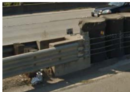
Figure 2: Backside of REACT 350 attenuator.
