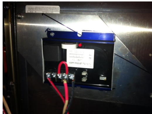
Figure 73: Physical Mounting for Low Voltage Disconnect.
