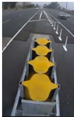
Figure 27: "Site C" with installed delineators.
