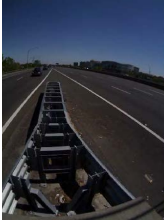
Figure 12 Daytime view of Smart Cushion installation
