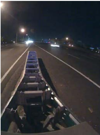
Figure 13: Nighttime view of the Smart Cushion installation.
