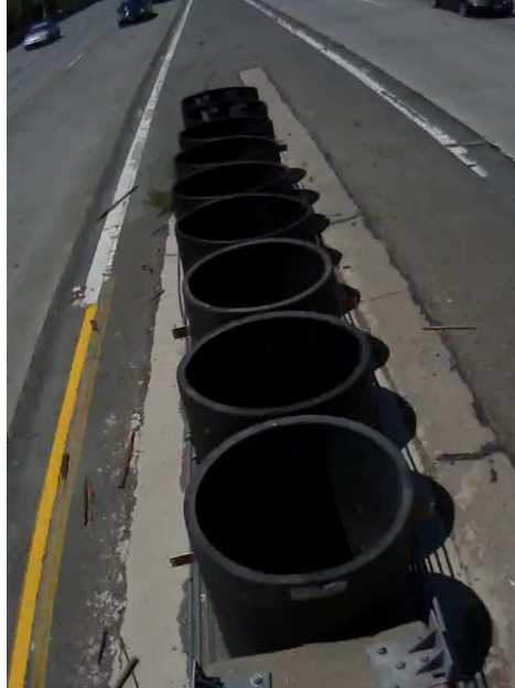
Figure 5: Daytime view of REACT350 attenuator.
