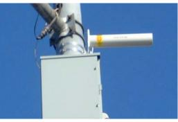
WLAN antenna and equipment mounted at intersection (Photo credit: Steve Gota, LACMTA)
