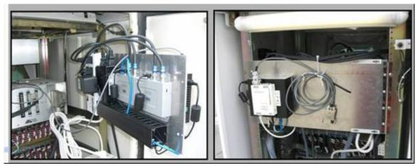
Figure 4-14: Front and Rear Views of Bridge/AP Intersection Panel
