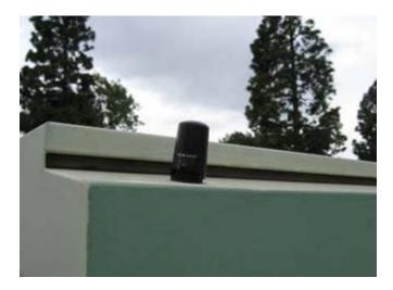
Figure 4-16: Typical WLAN Client Antenna Installation
