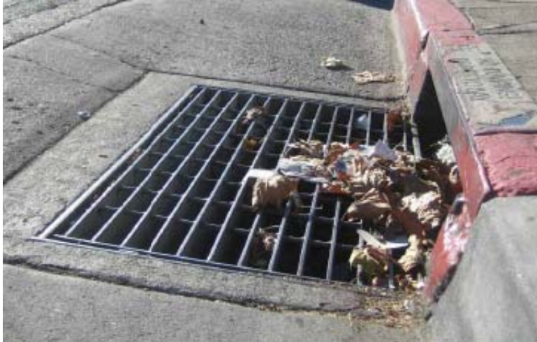
Figure 28 Storm Drain in front of Station #1
