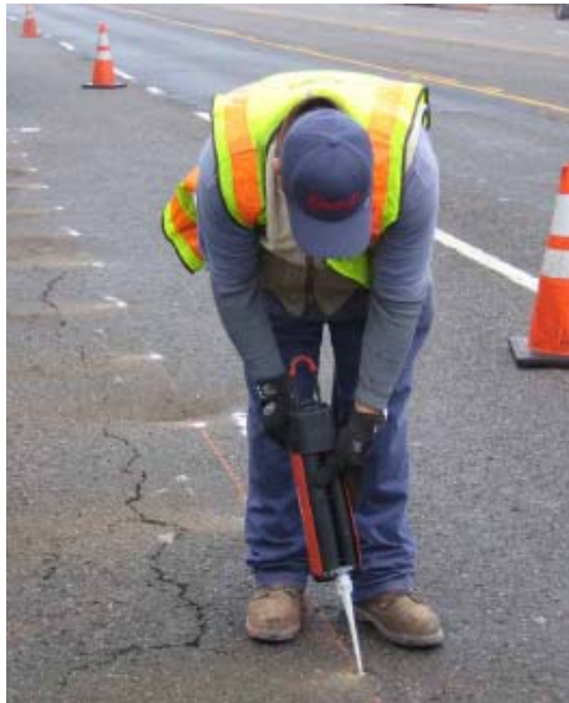
Figure 22 East 14 th Street. Installation: Sealing Magnets
