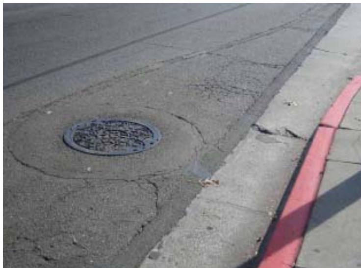
Figure 29 Utility access cover in front of Station #1
