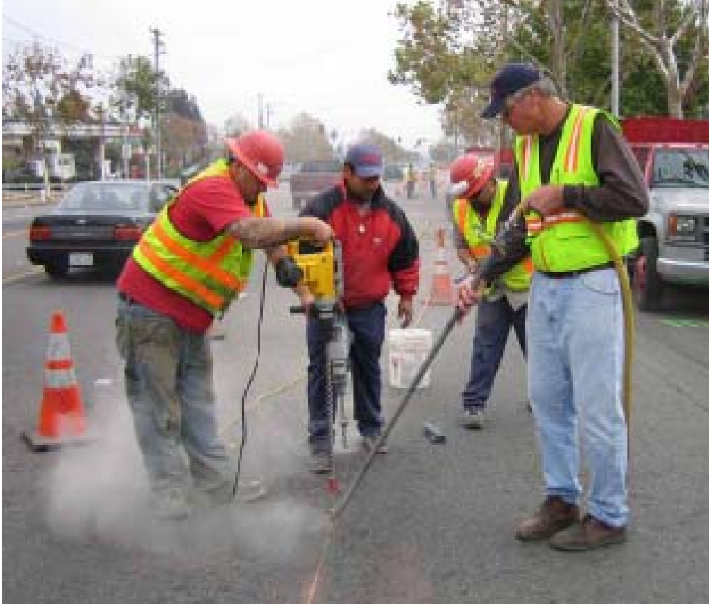
Figure 23 East 14 th Street. Installation: Two Team Installation (Drilling, Cleaning Holes and Placing Magnets)
