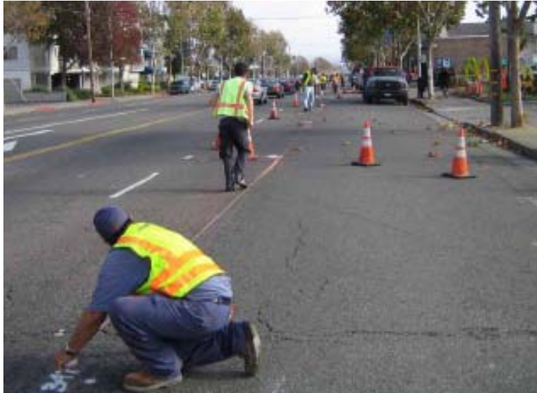
Figure 18 East 14 th Street. Installation: Chalk Line Based on 10m Survey Marks
