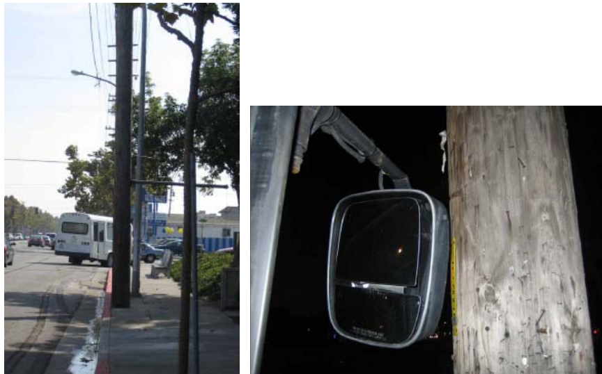
Figure 25 Utility Pole near Station #1 (right: 6" to curb; left: bus mirror next to pole when the bus is 20 cm to the curb)
