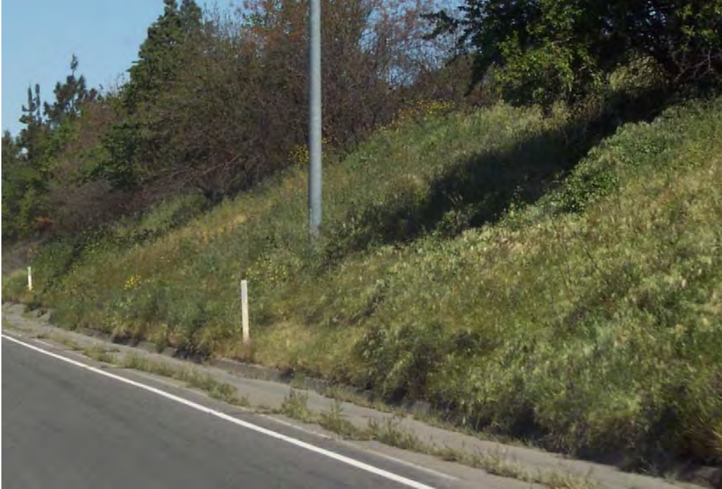
Figure 2.6 Urban Vegetation Overhanging Roadway and Sprouting in Crack
