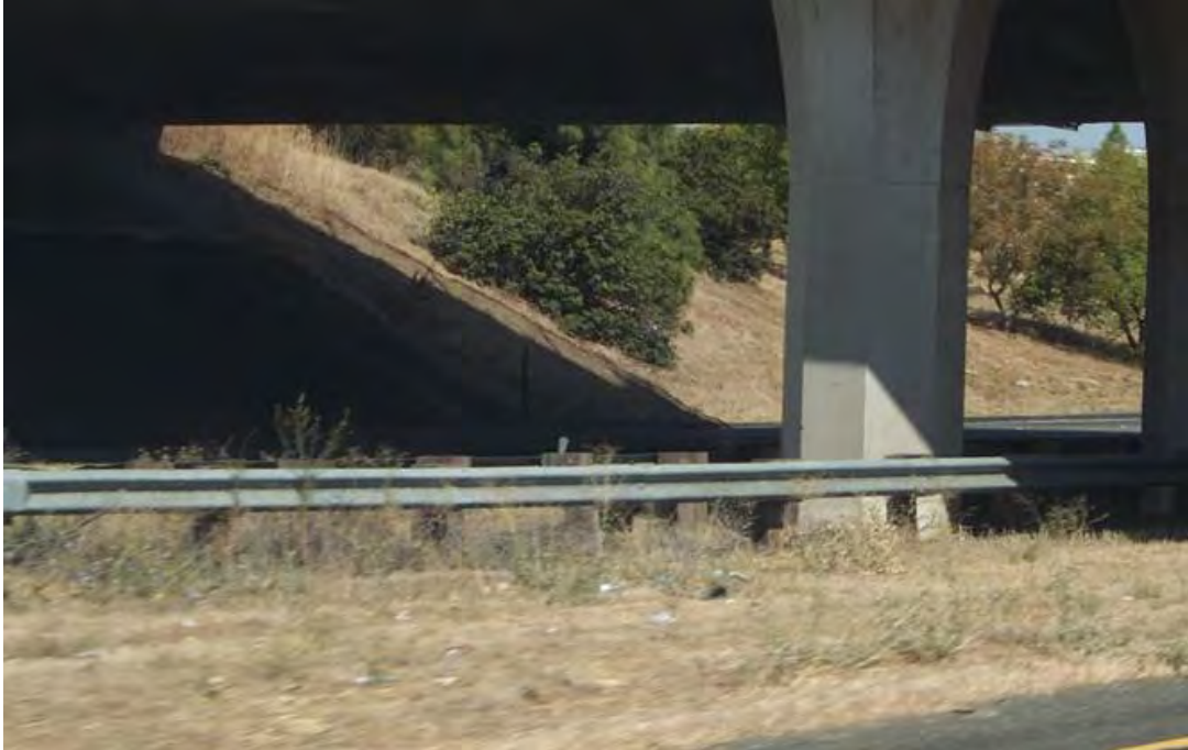
Figure 1.1 Guardrail around Overpass (Picture from [2])
