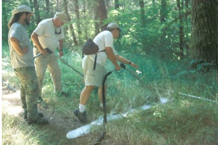
Figure 2-7 Workers applying Hot Foam [27]
