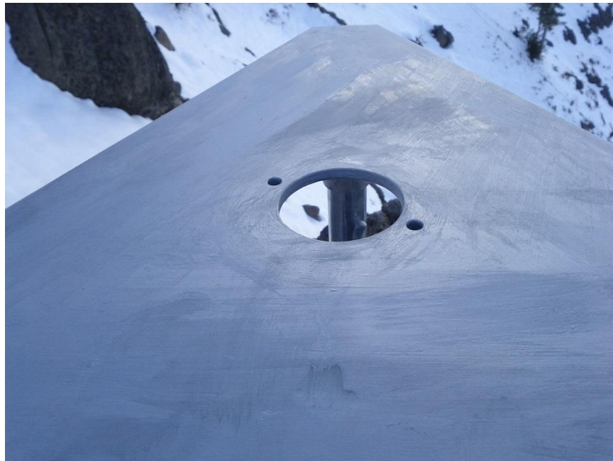
Figure C.11: The top plate with mounting for the wind generator mast
