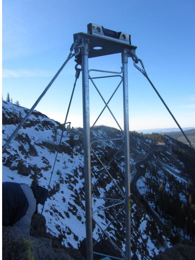
Figure 3.8: A view of the tower and top plate
