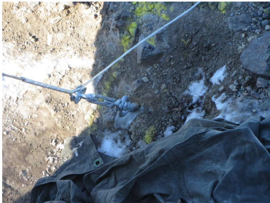
Figure C.7: A close-up of the north tower anchor
