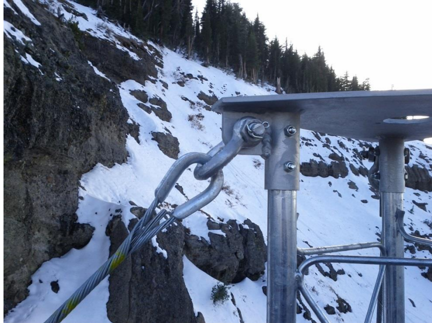
Figure C.10: A close-up of the anchor plate and guy wire attachment
