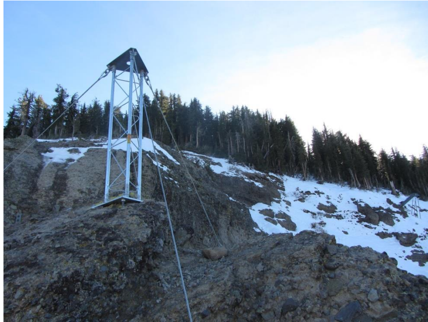
Figure 3.7: The south view of the final site's tower installation
