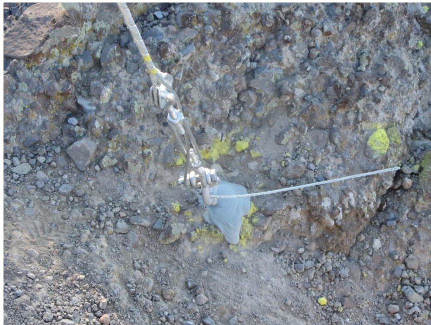
Figure C.5: A close-up of the southwest tower anchor
