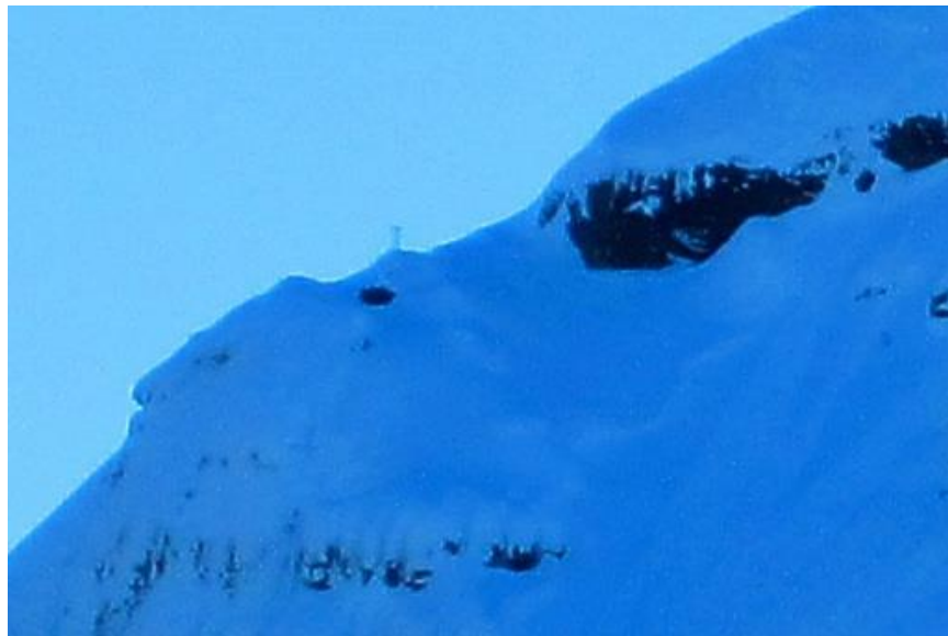
Figure B.2: Winter 2014 close-up of site installation. The tower is visible near the image center.
