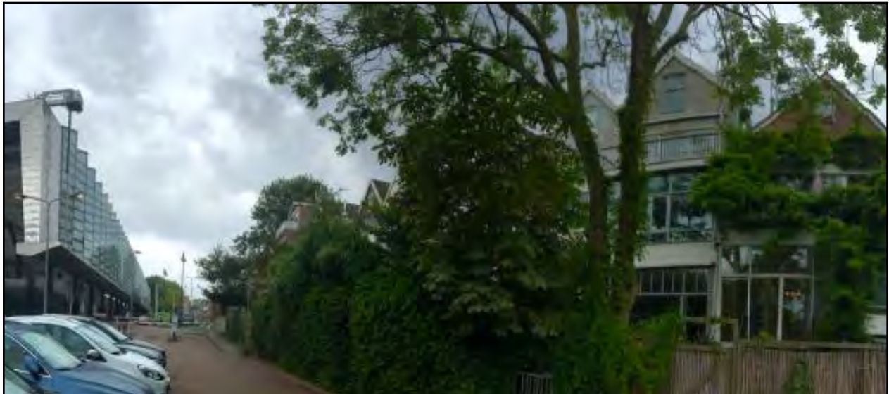
Figure 47. Residential Buildings Facing the Station's Northern Façade
