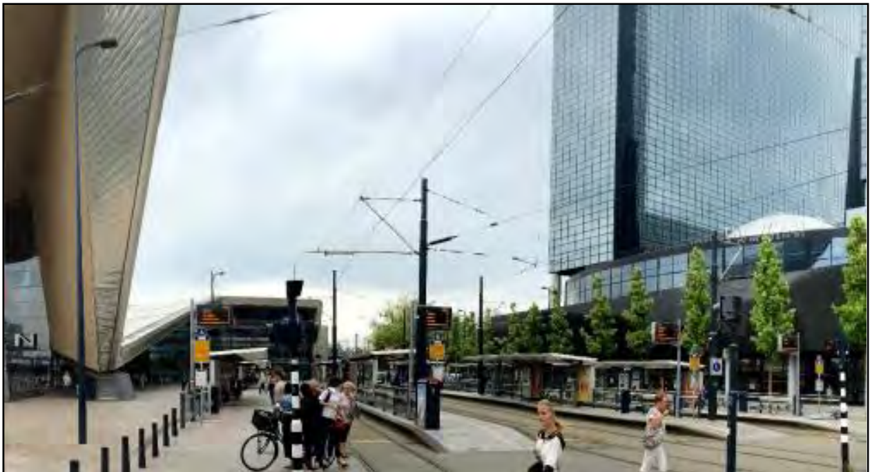
Figure 50. Multiple Tram Lines Now Converge on the East Side of the Station
