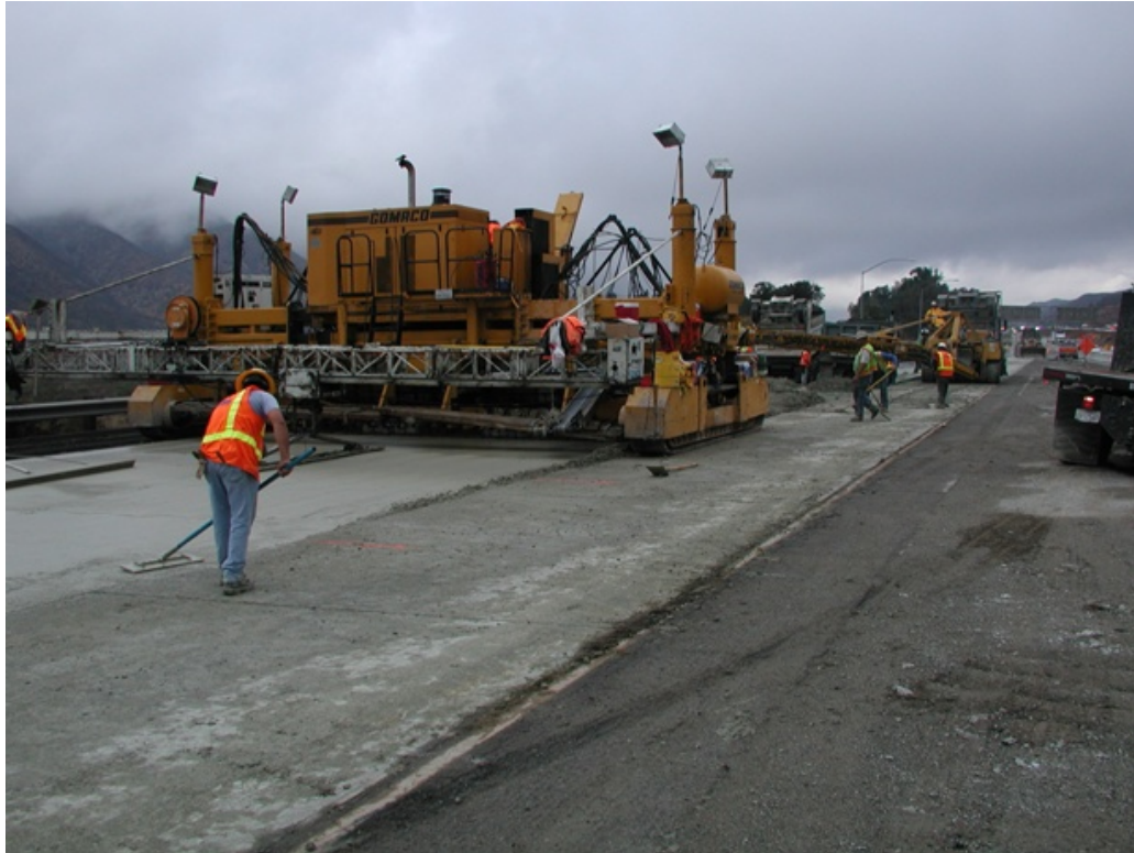
Figure 15: PCC slab paving.
