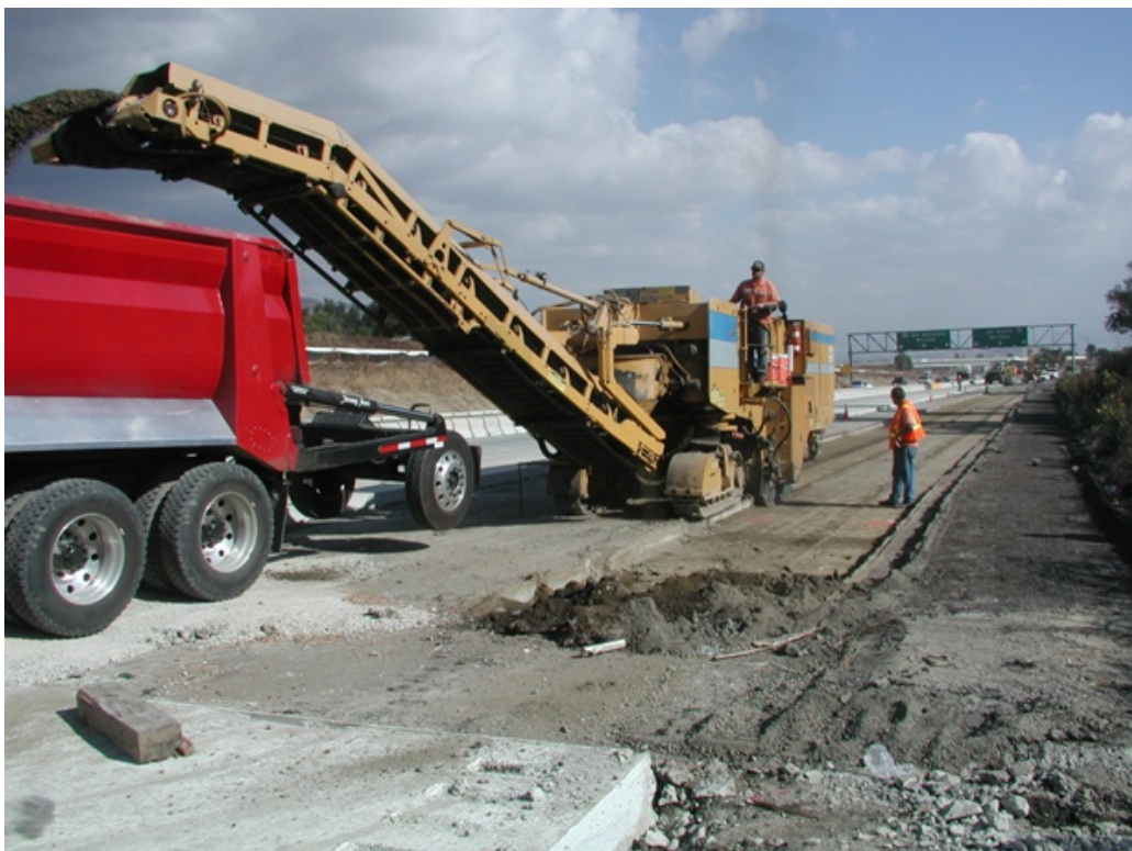
Figure 14: Milling of base.
