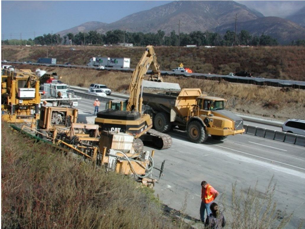
Figure 13: Demolition of PCC slab.
