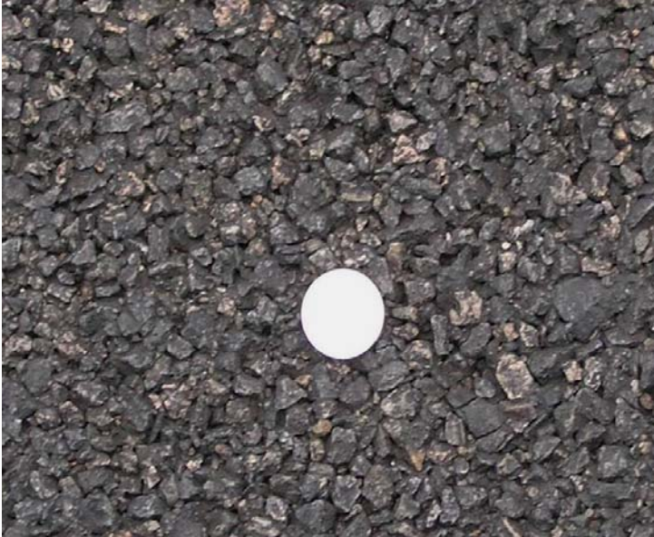
Figure 12: Open-graded asphalt concrete (OGAC).
