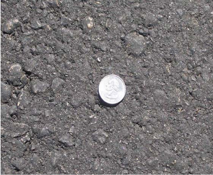
Figure 11: Dense-graded asphalt concrete (DGAC).
