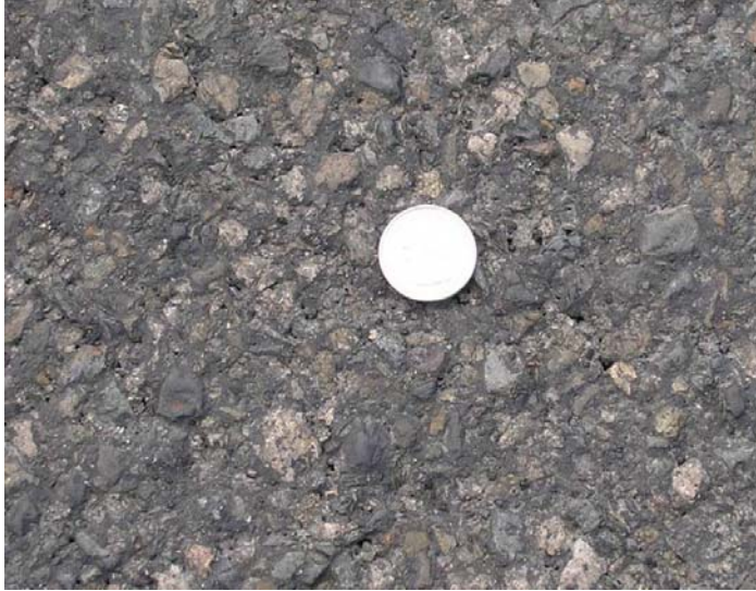
Figure 15: Rubberized gap-graded asphalt concrete (RAC-G).
