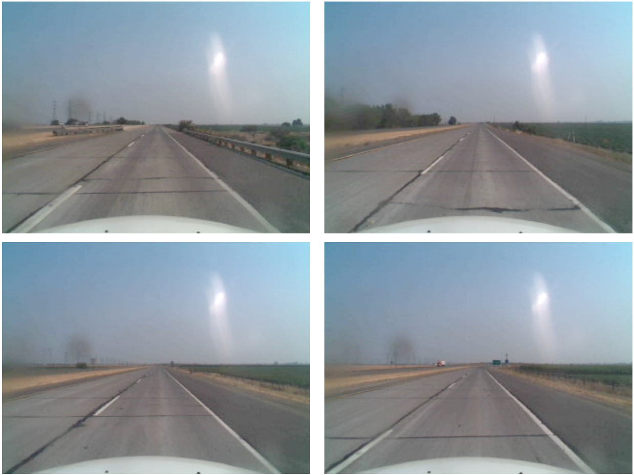
Figure B.1. View of segments A, B, C, and D on BD pavement.
