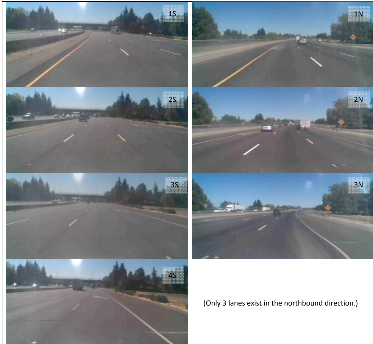
Figure A.18: Images of the pavement in every lane as seen from testing car, August 2008.
