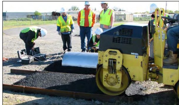
Figure 3.5: Test section compacting prior to sampling.
