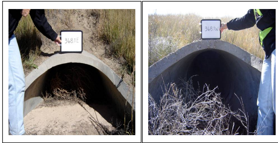
Figure 14. View of both entrances of R368.1; 52 x 104 cm (20.5 x 41 in; height x width) at eastbound entrance (left) and 93 x 118 cm (36.5 x 46.5 in) at westbound entrance (right).
