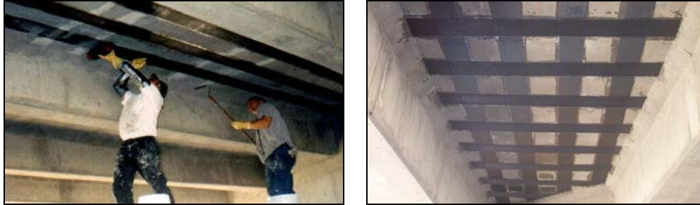
Figure 6.8. Wet Lay-up Construction
