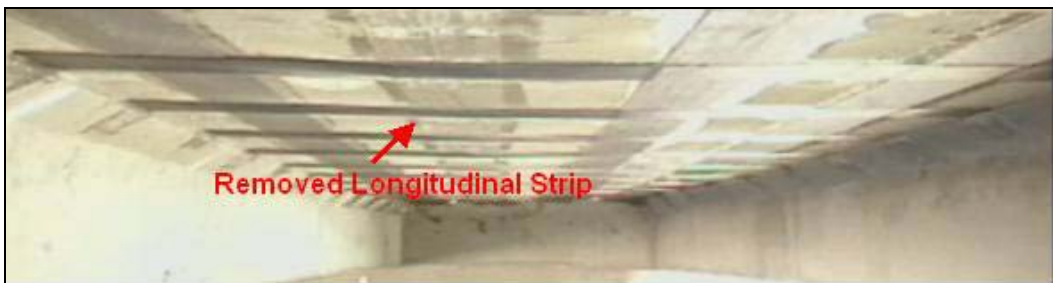
Figure 10.5. Removal of Longitudinal CFRP Strip in Location S9B5
