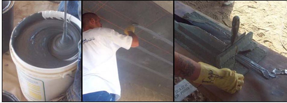
Figure 6.10. Mixing and Application of Adhesive
