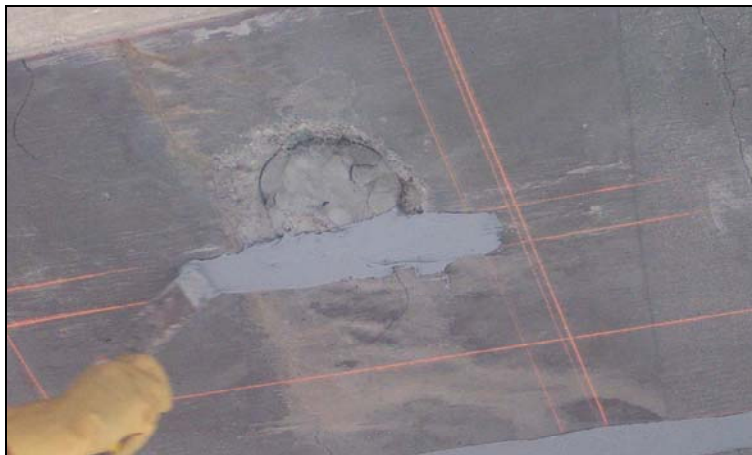
Figure 7.6. Cavity in Bay 9-1 Filled with Epoxy Adhesive
