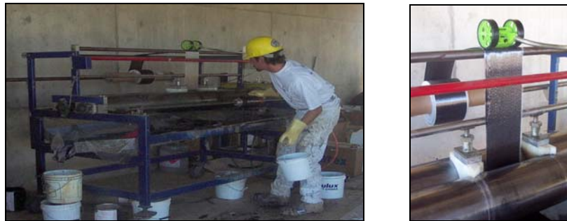
Figure 6.9. Impregnator for Wet Lay-up CFRP
