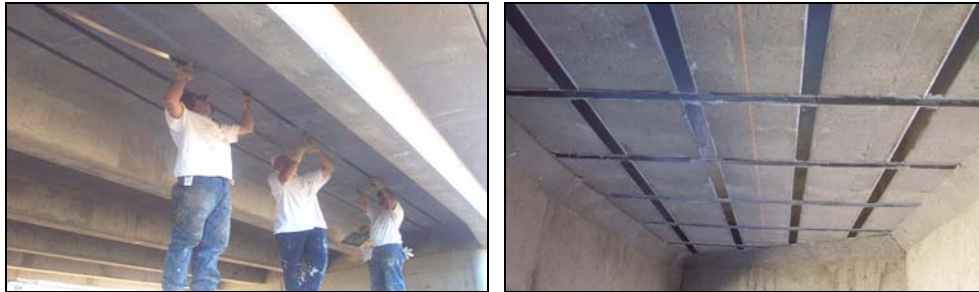
Figure 6.11. Pultruded Strip Construction
