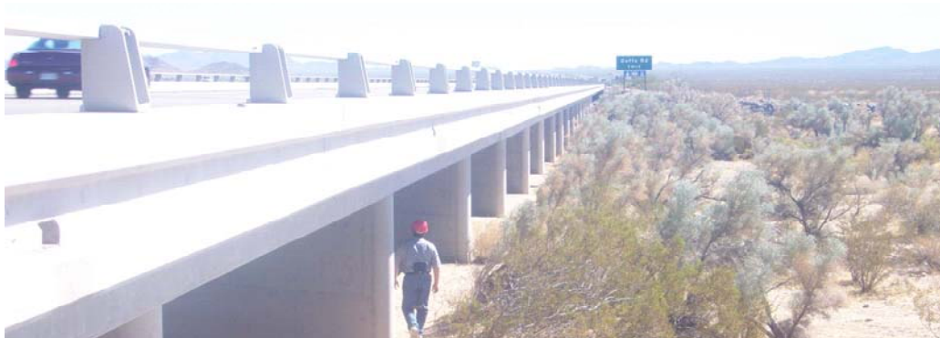
Figure 5.2. Watson Wash Bridge
