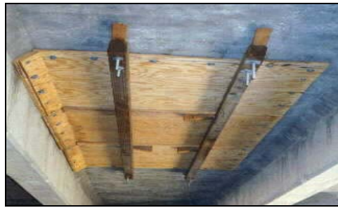
Figure 6.4. Caltrans Repair at Location S8B4
