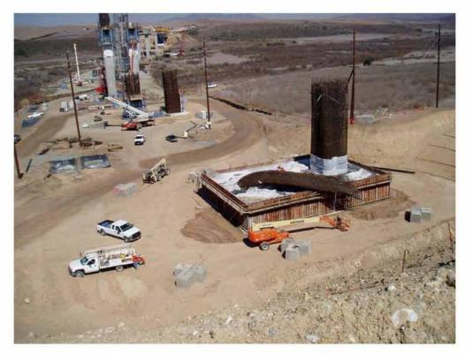
Figure 1.6: Bridge Column Rebar Cage after Collapse in Sweetwater River Connection
