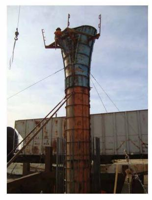
Figure 2.18: Column Forms with Temporary Support installed
