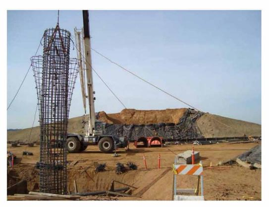
Figure 1.10: Bridge Column Rebar Cage being held by a Crane
