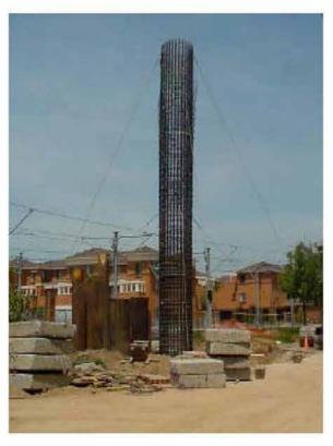
Figure 2.25: Column Rebar Cage with Two Levels of Four Guy cables
