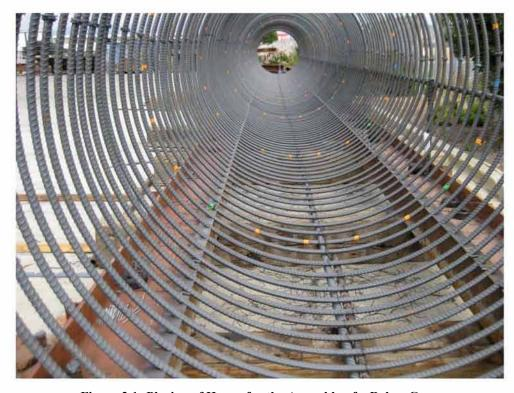
Figure 2.1: Placing of Hoops for the Assembly of a Rebar Cage
