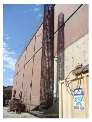
Figure 3.51: Specimen II standing without any Temporary Support
