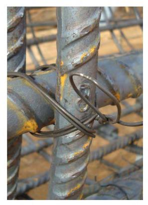
Figure 2.11: Figure-Eight Tie Wire Connection
