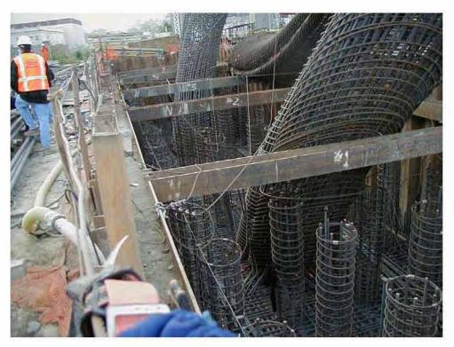
Figure 1.3: Close-up of the footing for both Columns in Bent 7 of Carquinez Bridge
