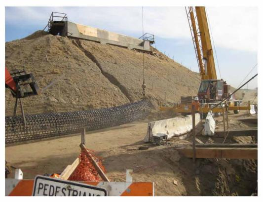
Figure 2.19: Column Rebar Cage being lifted by the Crane with the help of a Forklift
