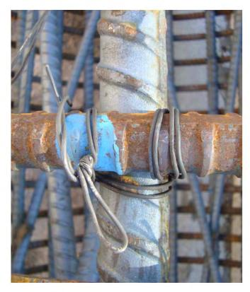
Figure 2.10: Wrap-and-Saddle Tie Wire Connection
