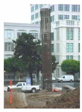
Figure 1.8: Column Rebar Cage supported by four Guy cables in bent 23 of SFOBB West Approach
