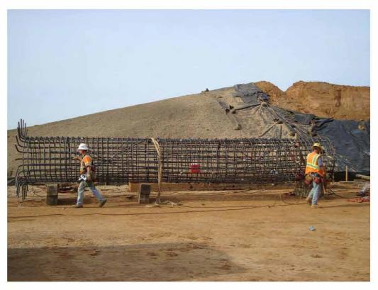
Figure 2.21: Rebar Cage with two X-braces ready to be lifted
