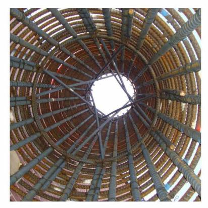
Figure 2.16: Detail of Internal Square Brace
