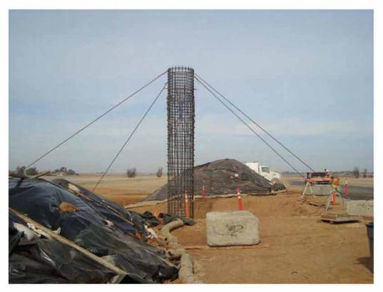
Figure 2.27: Column Rebar Cage with four guy cables
