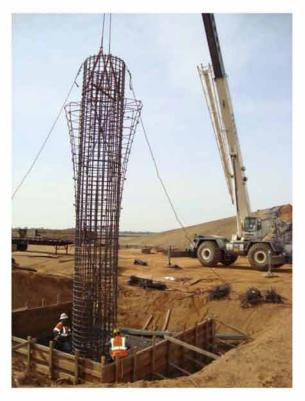
Figure 2.23: Column Rebar Cage being Attached to the Bottom Mat of the Footing
