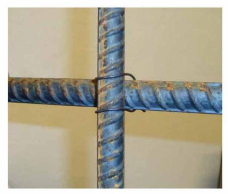
Figure 2.8: Single-U Tie Wire Connection
