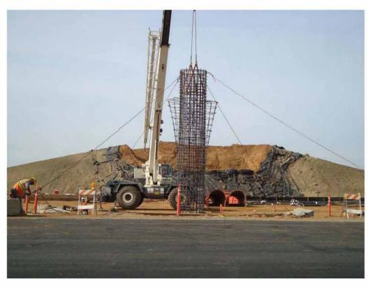
Figure 2.24: Column Rebar Cage being guyed at four locations
