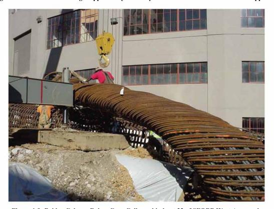
Figure 1.9: Bridge Column Rebar Cage Collapsed in bent 23 of SFOBB West Approach
