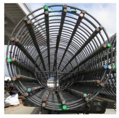
Figure 2.2: Pick-up Bars in a Column Rebar Cage
