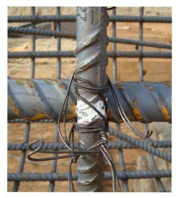
Figure 2.12: Column-Tie Connection
