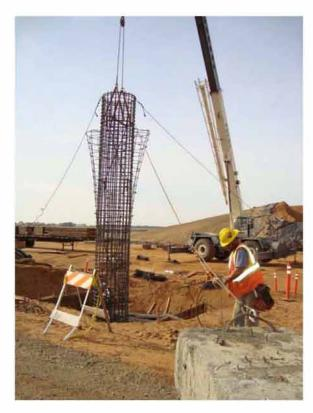
Figure 2.26: Remove of slack in guy cables
