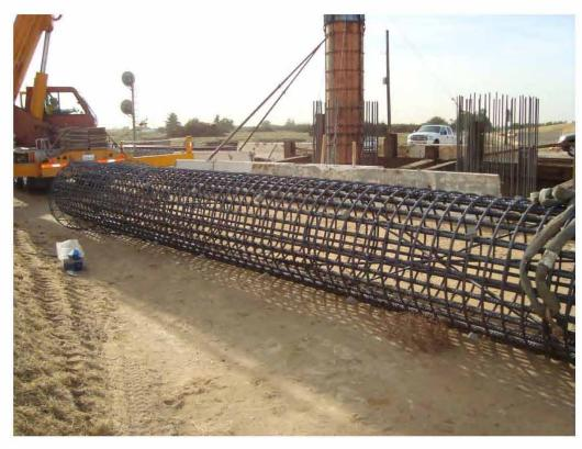
Figure 2.17: Rebar Cage with two X-braces ready to be lifted
