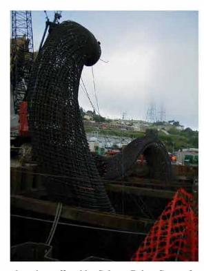
Figure 1.4: Bending and torsion suffered by Column Rebar Cages after collapse in Bent 7 of Carquinez Bridge
