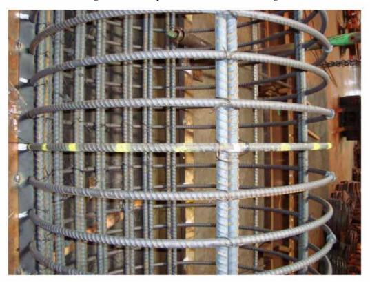
Figure 2.3: Template-hoops in a Column Rebar Cage
