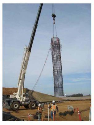
Figure 2.22: Rebar Cage being swung into the location of the footing
