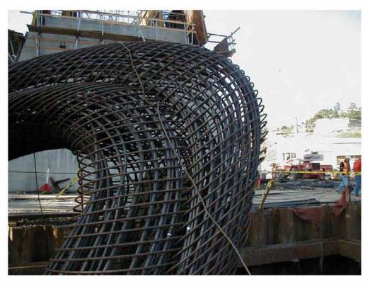
Figure 1.5: No presence of Internal Braces in Bridge Column Rebar Cage in Bent 7 of Carquinez Bridge
