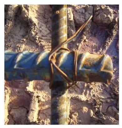
Figure 2.9: Double-U Tie Wire Connection
