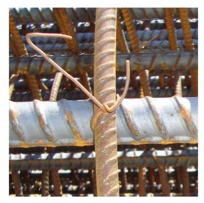
Figure 2.6: Single-Snap Tie Wire Connection
