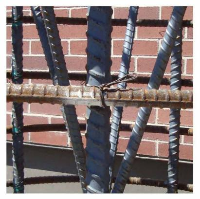
Figure 2.7: Double-Snap Tie Wire Connection
