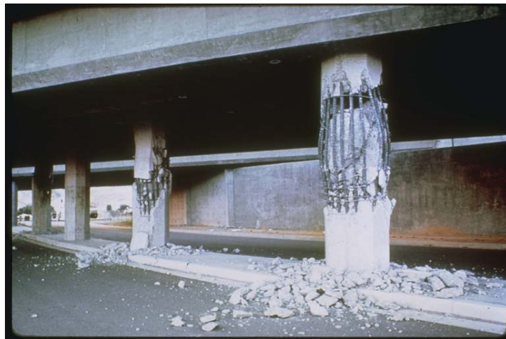
Figure 3.5: Shear failure in bridge columns a) at the intersection of Interstate 5 and 210, and b) of Foothills Freeway Overpass, during the San Fernando earthquake
