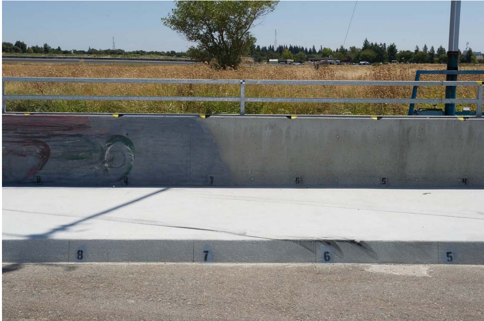
Figure 3-13 – Type 732SW bridge rail face after 130MASH3C13-02
