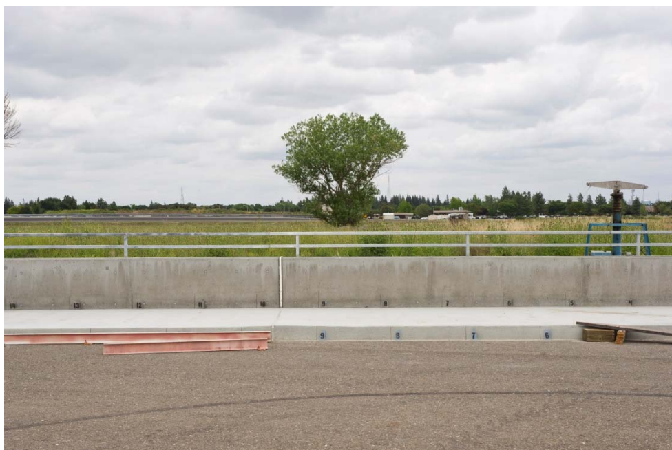
Figure 3-1 – Test article prior to Test 130MASH3P13-01
