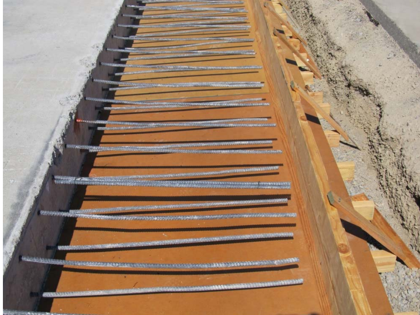
Figure 2-2 – New rebar spliced with existing rebar for new bridge deck
