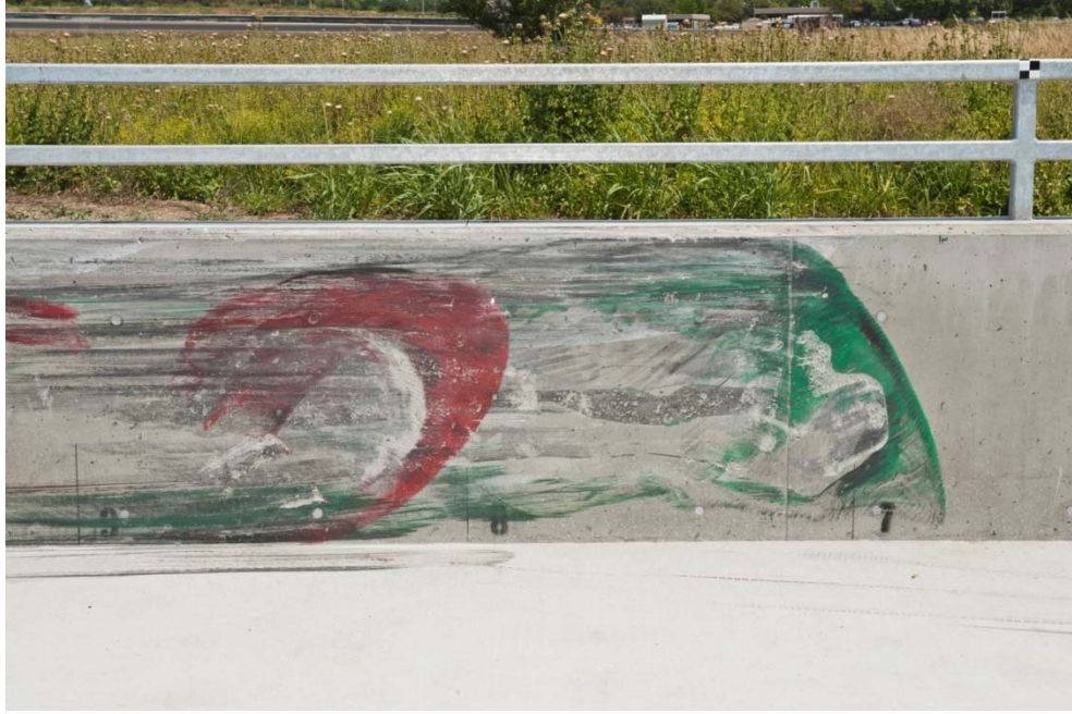
Figure 3-3 – Close-up of 732SW Barrier after Test 130MASH3P13-01
