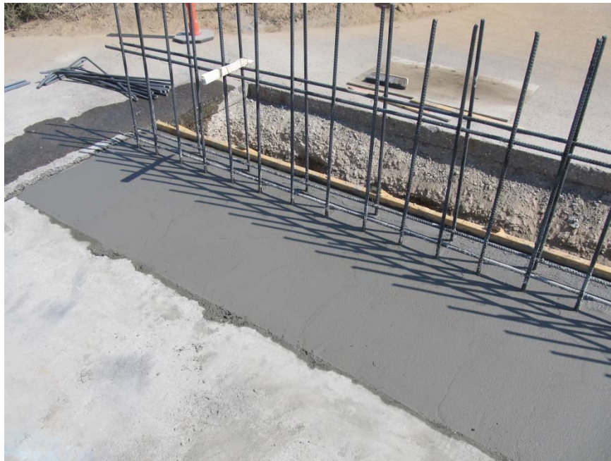
Figure 2-3 – New bridge deck in place for Type 732SW bridge rail
