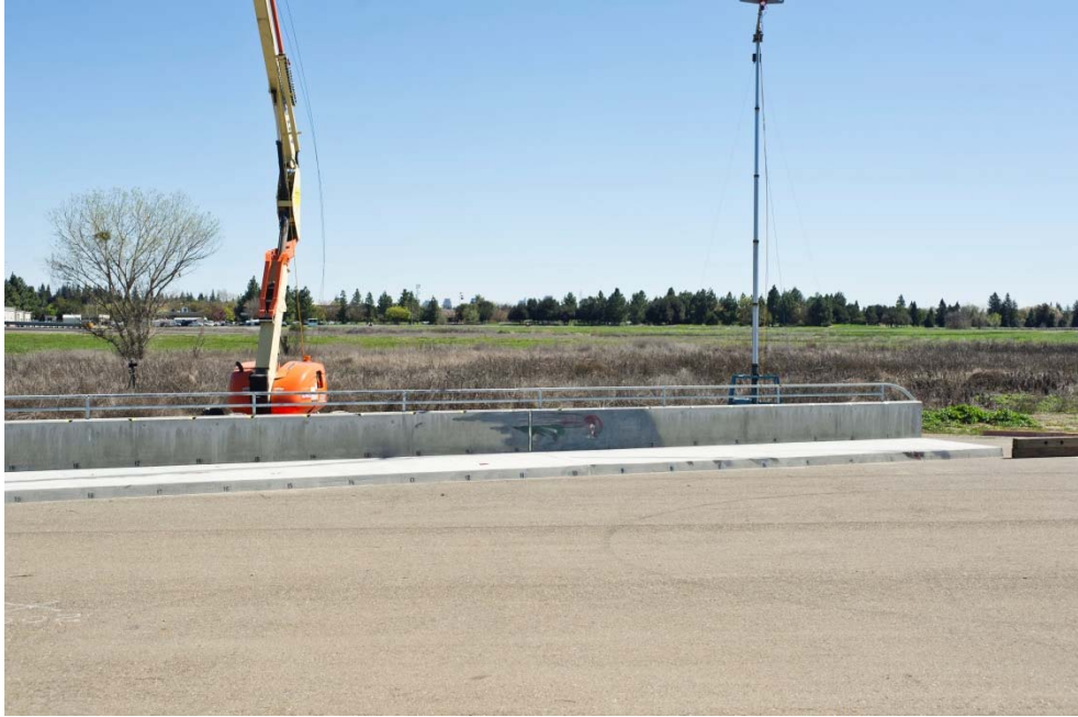
Figure 3-24 – Type 732SW bridge rail face after Test 110MASH2C14-01
