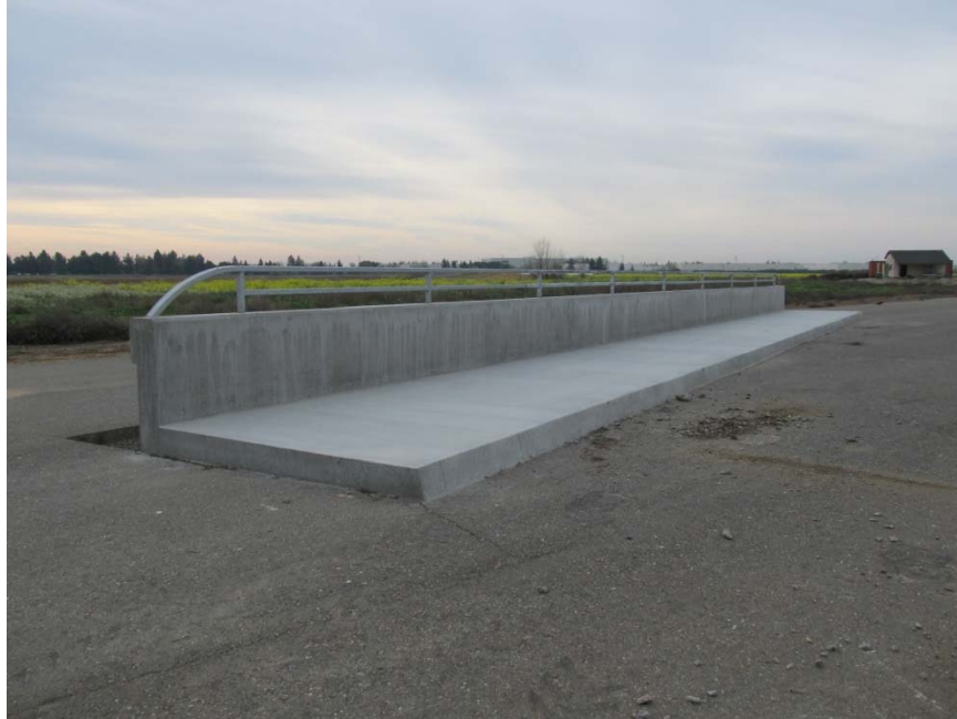
Figure 2-6 – Type 732SW with the steel handrail in place
