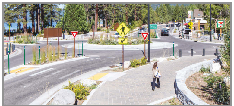
State Route 28 was converted from four lanes to three to accommodate new sidewalks, Class II bike lanes, and bus shelters. Two single-lane roundabouts were constructed to slow traffic.
