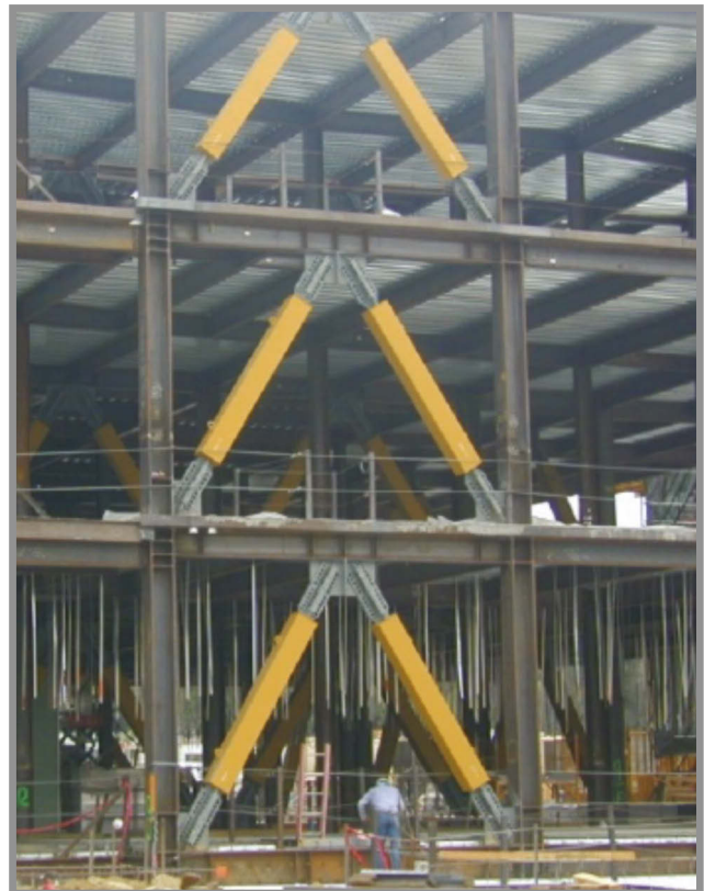
Typical BRB frames within a building structure
