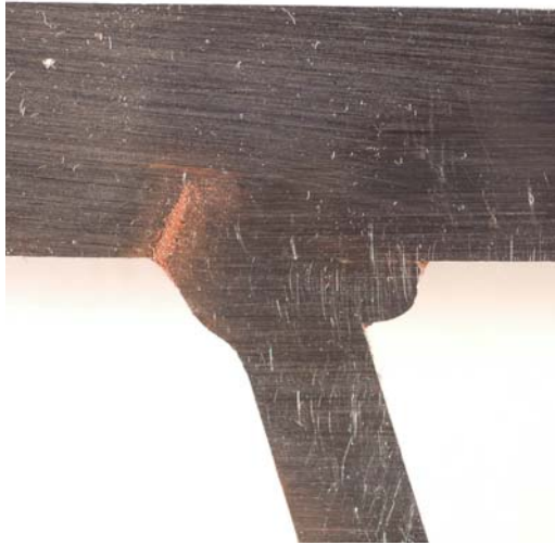
(a) Crack from Weld Toe
