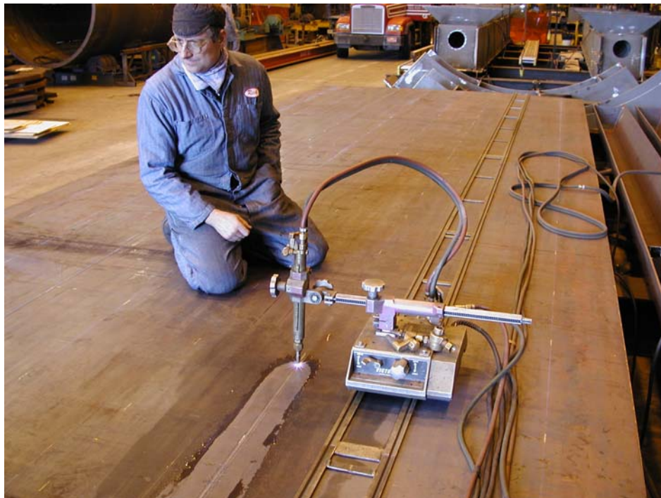
Figure 2.7 Heat Straightening Operation
