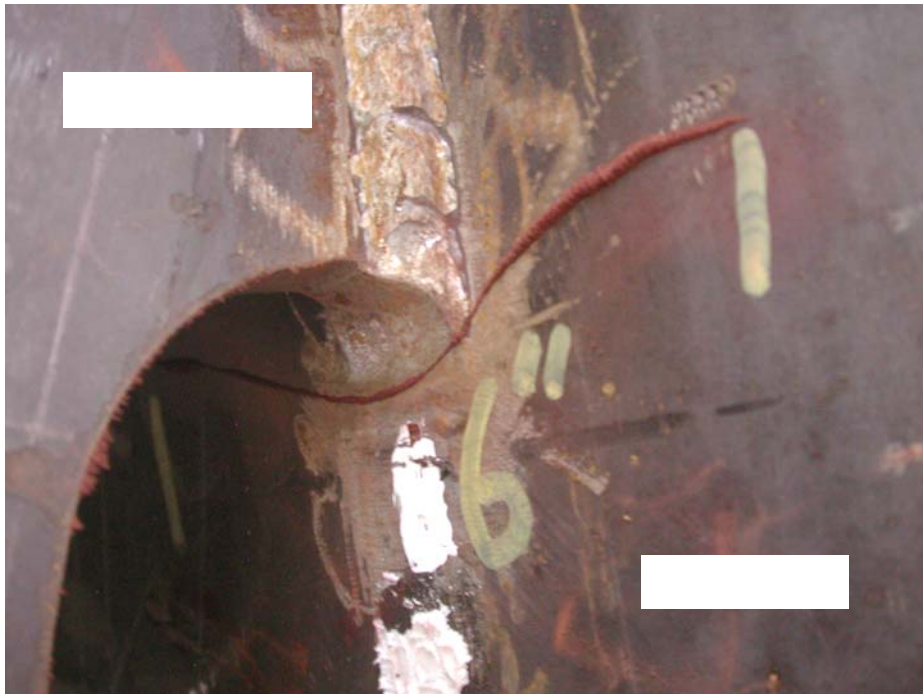
(b) View from Outside of Rib
