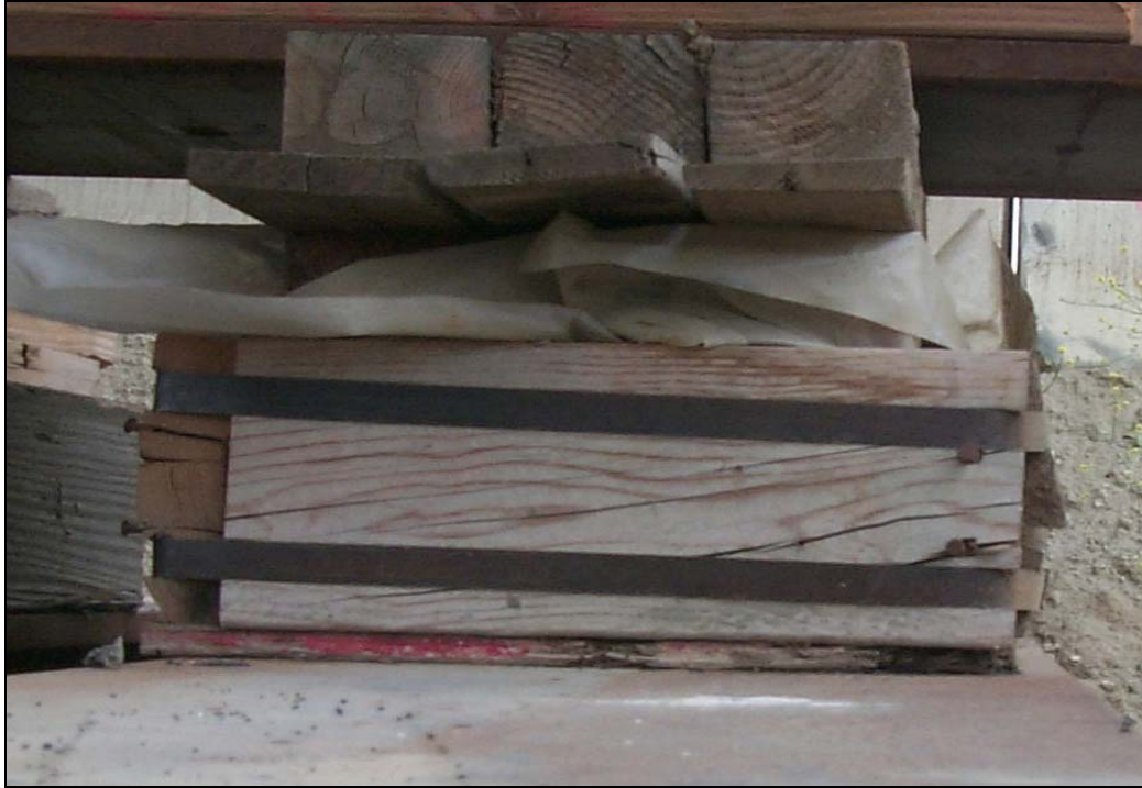
Figure 1.2: Close up of Sand-Jack in use.
