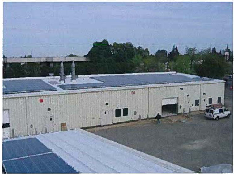
State Headquarters Materials and Testing Laboratory, Sacramento (Sacramento Translab)
