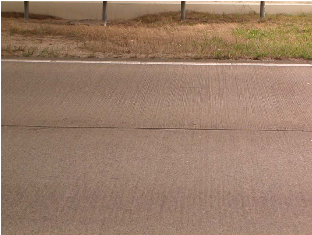
Figure 31: Photograph randomly textured PCC in the Netherlands on the A270 roadway (reference no. 33)
