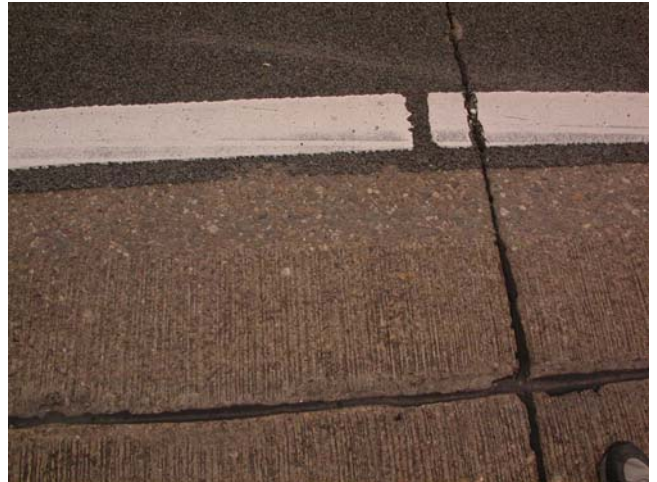
Figure 32: Photographs of epoxy and stone layer as applied to randomly textured PCC in the Netherlands on the A270 Roadway (reference no. 36)
