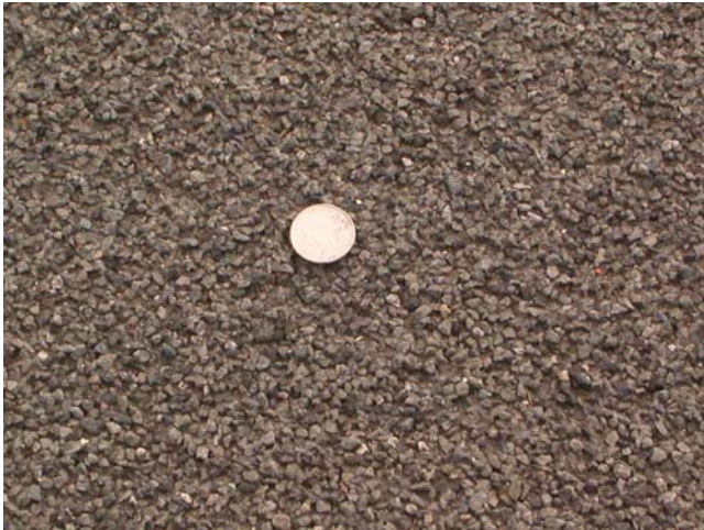
Figure 32: Photographs of epoxy and stone layer as applied to randomly textured PCC in the Netherlands on the A270 Roadway (reference no. 36)
