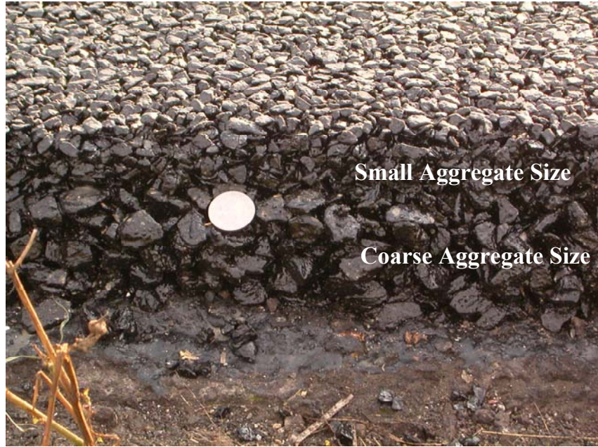
Figure 23: Photograph of typical double layer porous asphalt construction in the Netherlands
