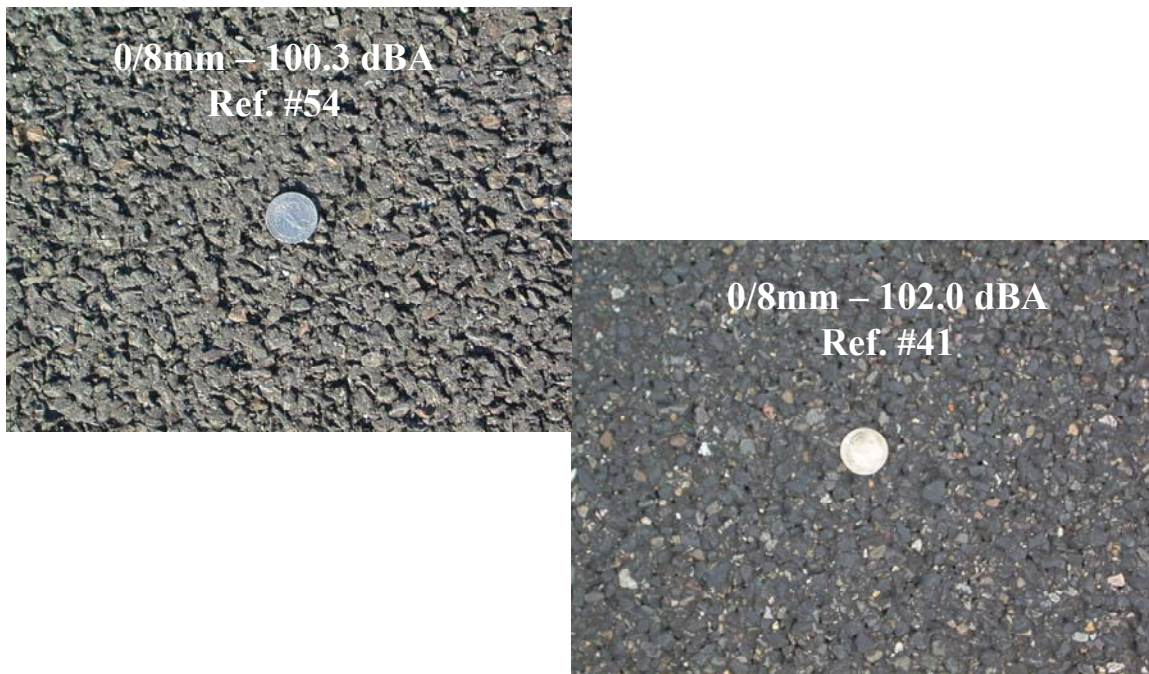
Figure 18: Photographs of two SMA surfaces containing narrower (a.) and wider (b.) ranges aggregate size resulting in different apparent surface roughness
