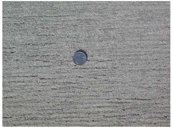
Figure 33: Photographs of cross-hatched grooved (reference no. 65) and smooth PI (reference no. 64) PCC surfaces at the Sperenberg test track
